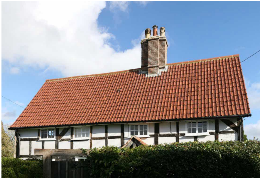
Figure 4 Western Elevation with slate tiles removed.
