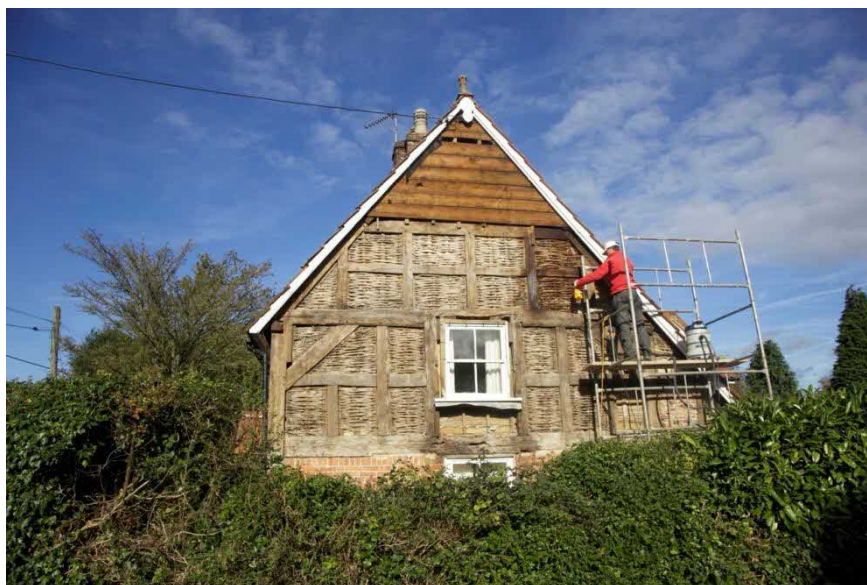
Figure 2 Renovation works in 2012.
