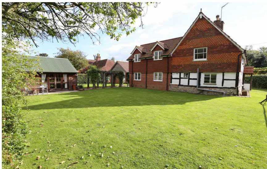
Figure 5 Northern Elevation showing tiles to older part of the house.
