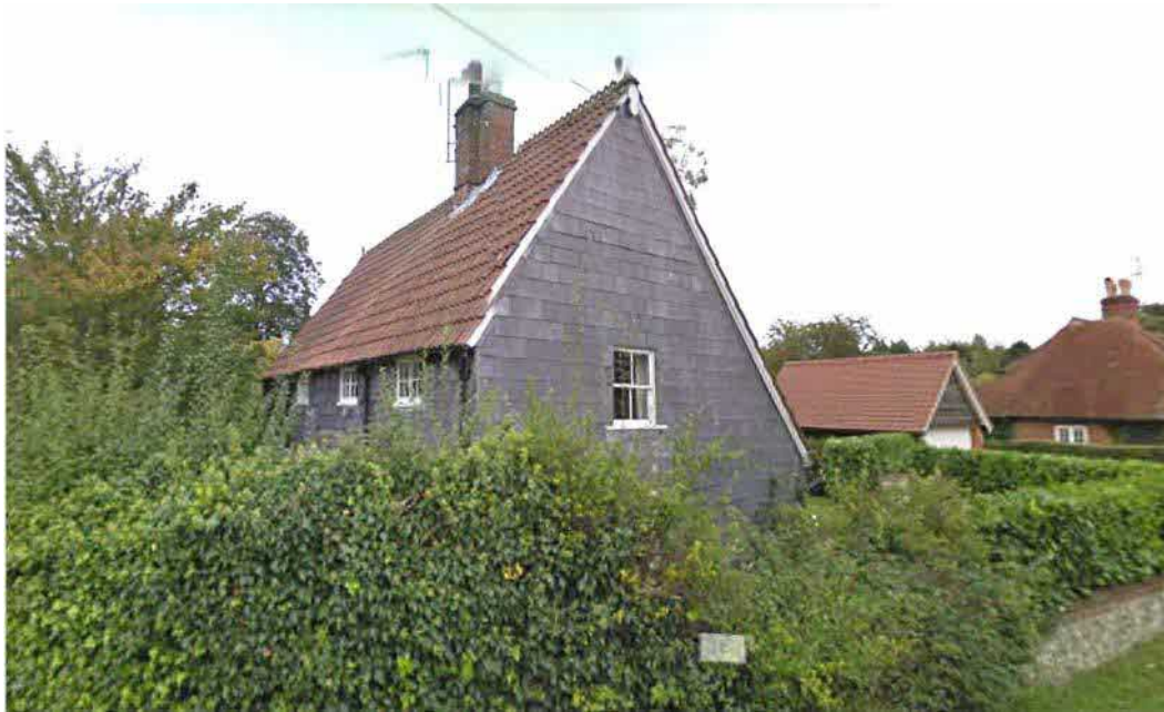
Figure 1 West Cross House prior to the removal of the slate hanging to the west and south elevations. © Google Maps
