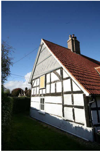
Figure 3 Southern Elevation with slate tiles removed and temporary measures in place.
