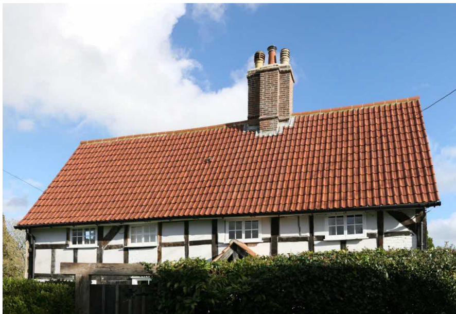
Figure 4 Western Elevation with slate tiles removed.
