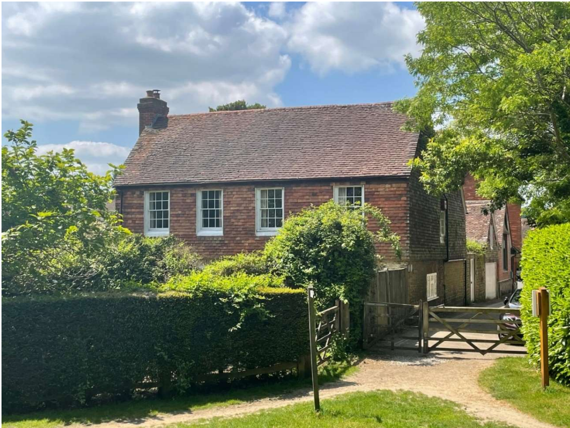
Front (East) Elevations taken from St Annes Hill
