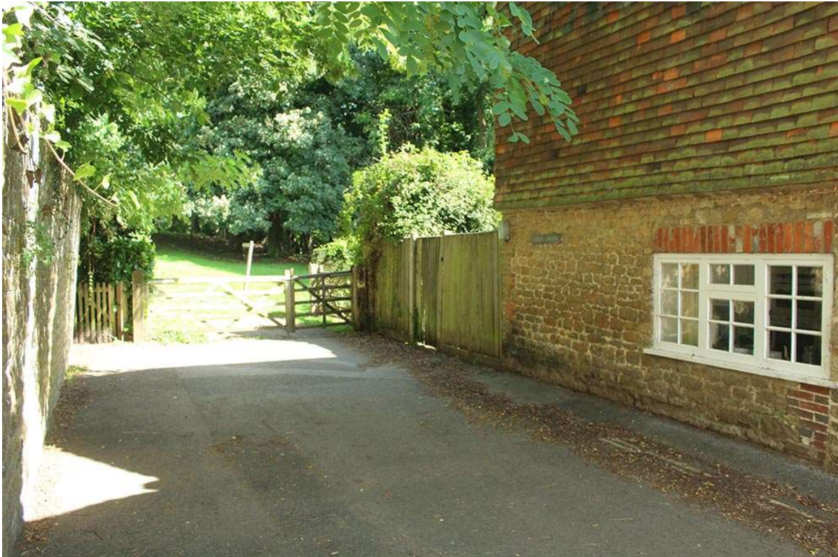
Figure 2 The existing entrance to the castle site (through the five-bar gate and adjoining pedestrian gate) looking eastwards along St. Ann's Hill, with Court Green to the right
