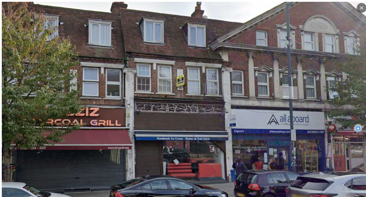
FIGURE 1: 226 STATION ROAD (CENTRE UNIT)
