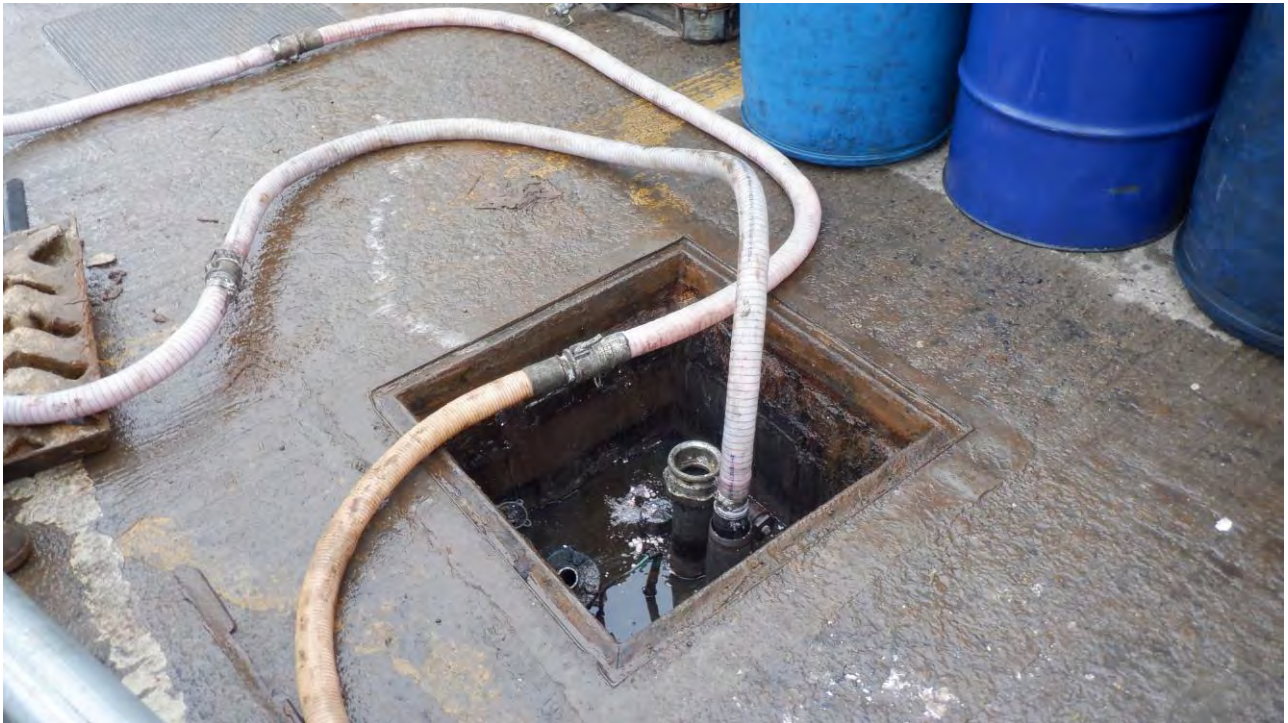
Photograph 3: Filling pipework attached to Tank 4.
