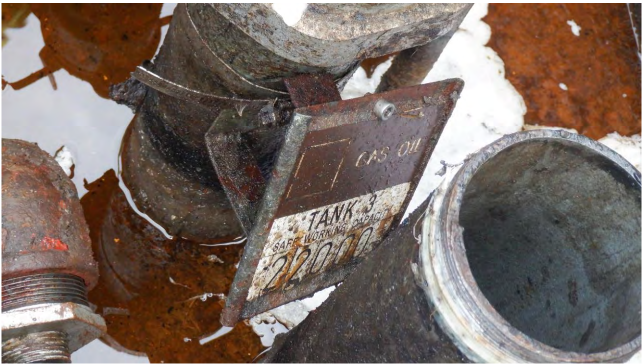
Photograph 7: Label on Tank 3 indicating 22,000 litre capacity.
