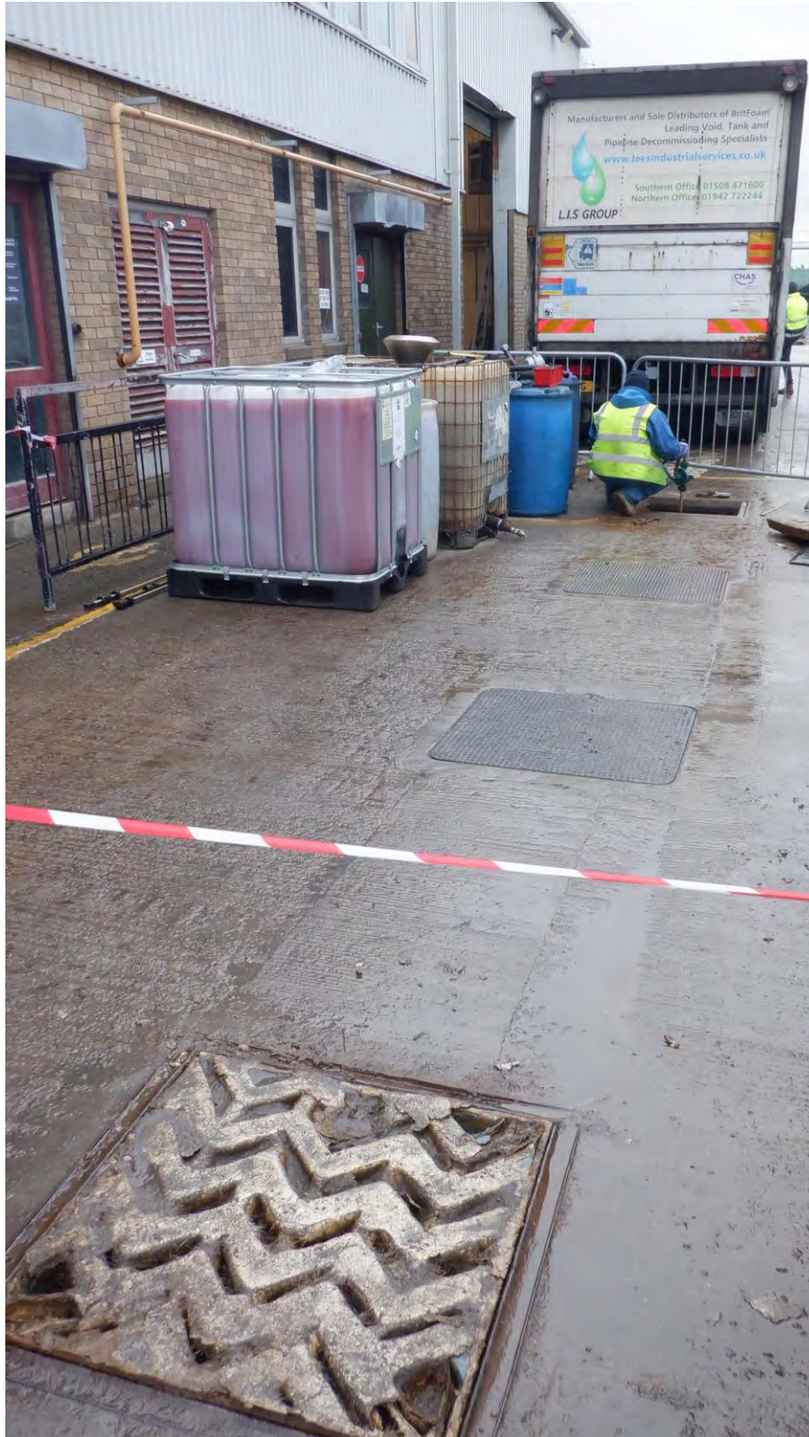
Photograph 1: WO Silmon emptying the last of Tank 4 (contents shown in IBC containers and barrels).
