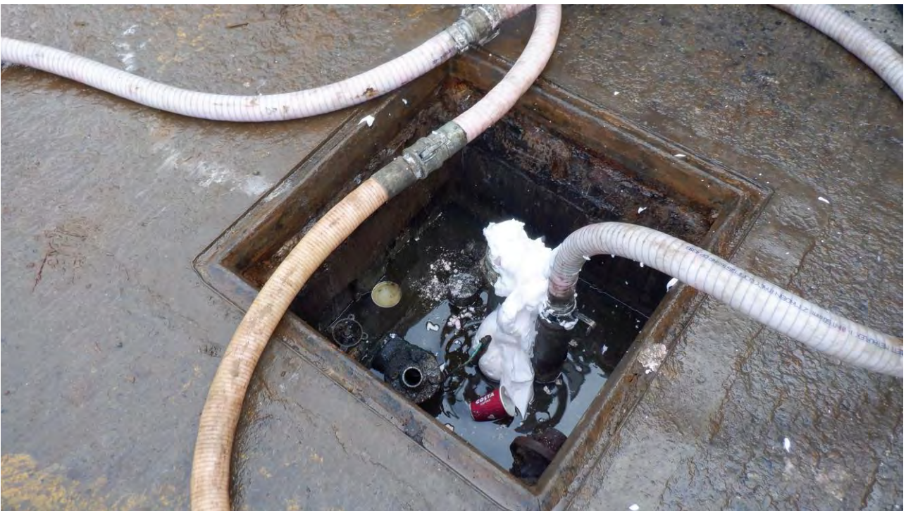
Photograph 5: Foam reaching surface level as tank is filled.
