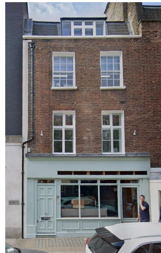
Existing Front façade from Eccleston Street
