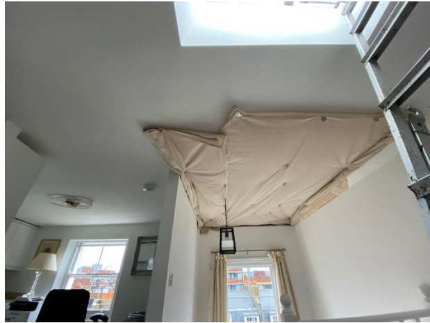
Figure 3: Fourth floor ceiling showing the position of the approved rooflight
