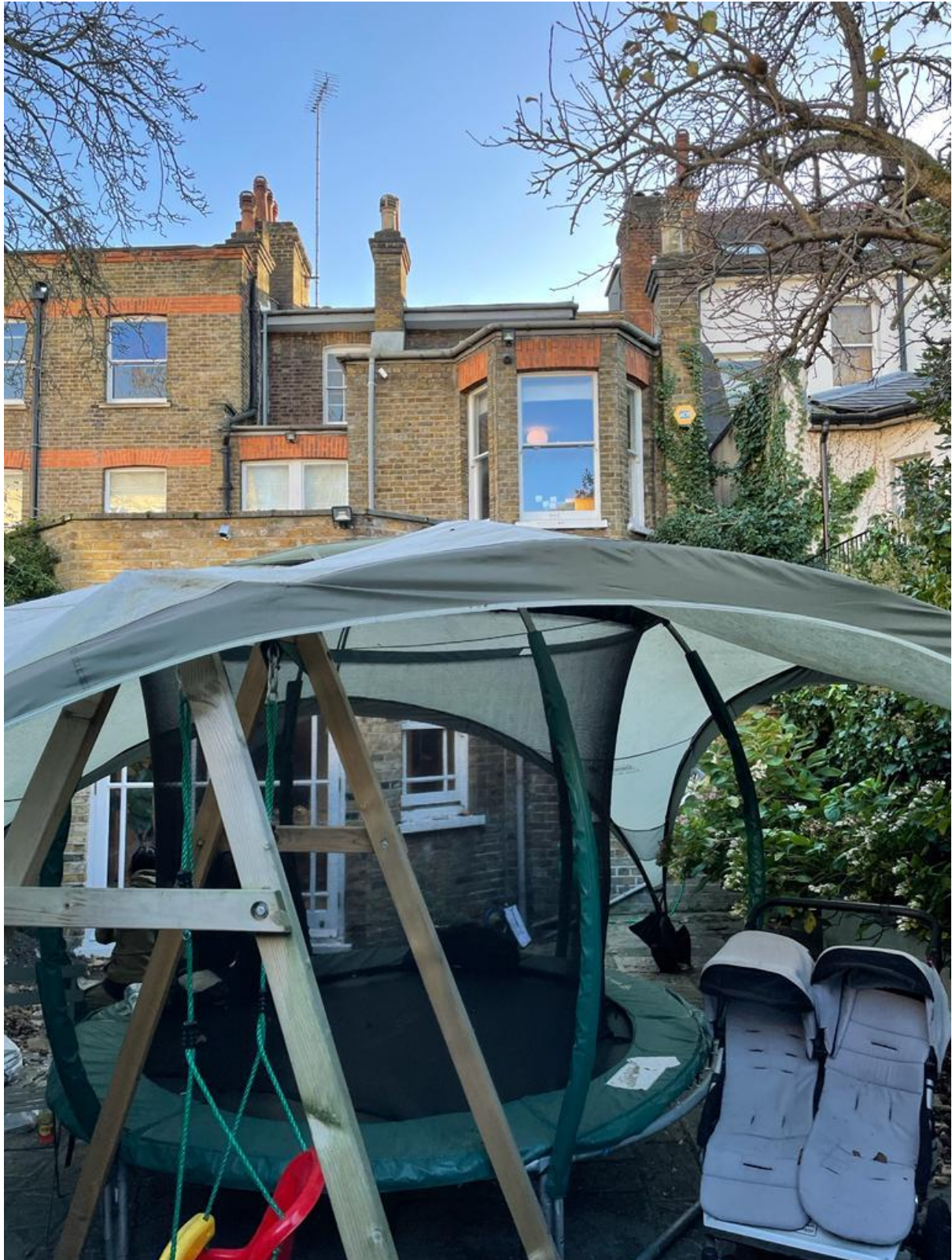
Photograph 11 – View overlooking the rear of the 3-storey building.
