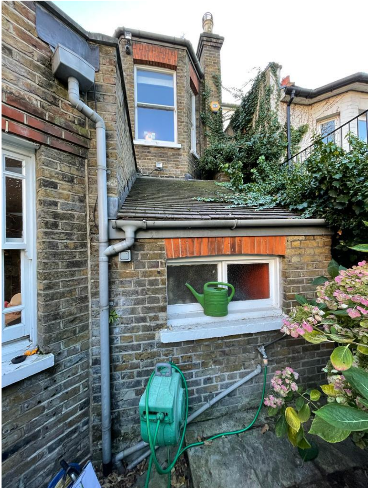
Photograph 15 – Rear of the building, viewing towards the south.
