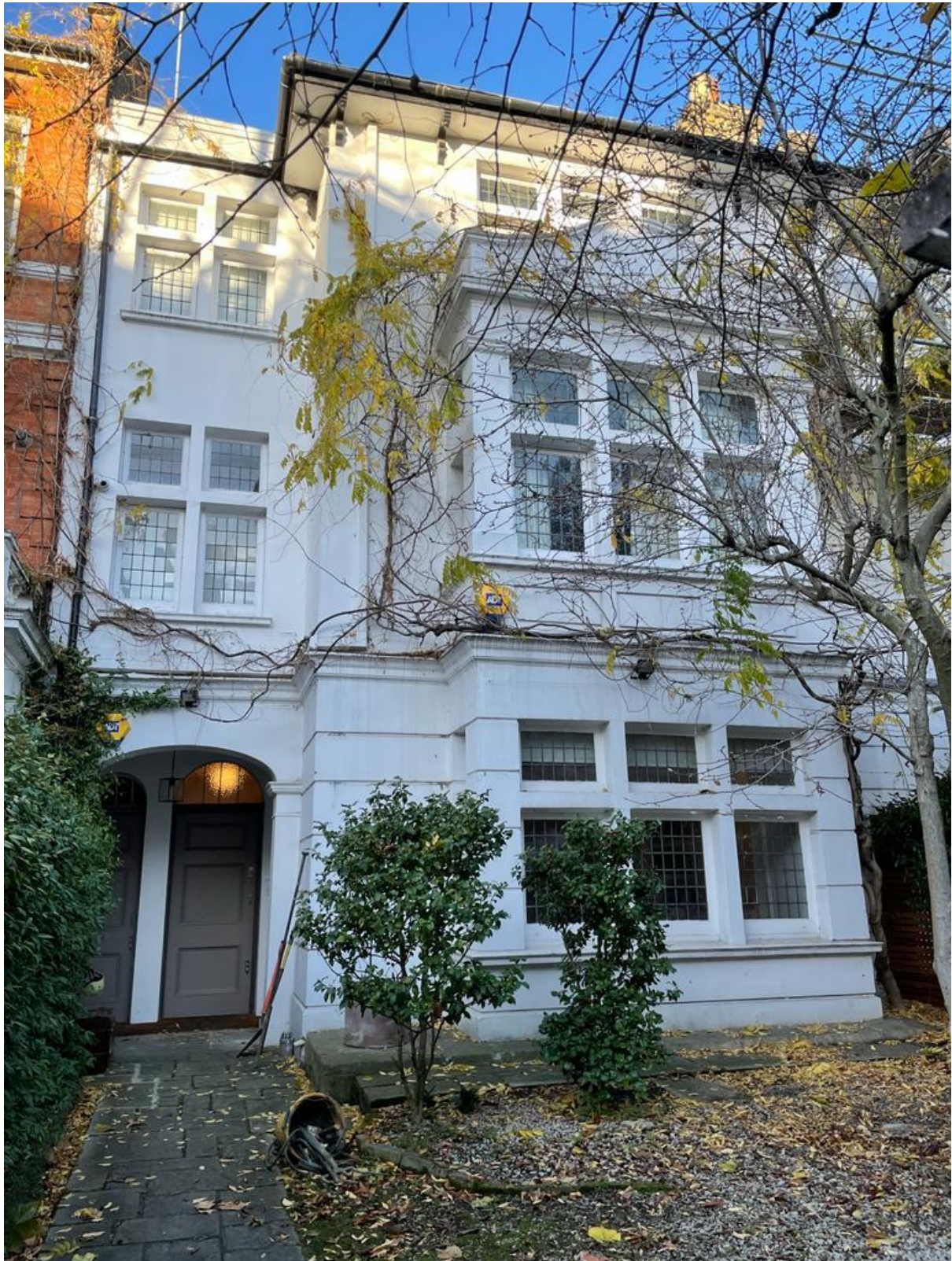
Photograph 1 – Front of the 3-storey residential terraced property in the south of the site, viewing towards the north.
