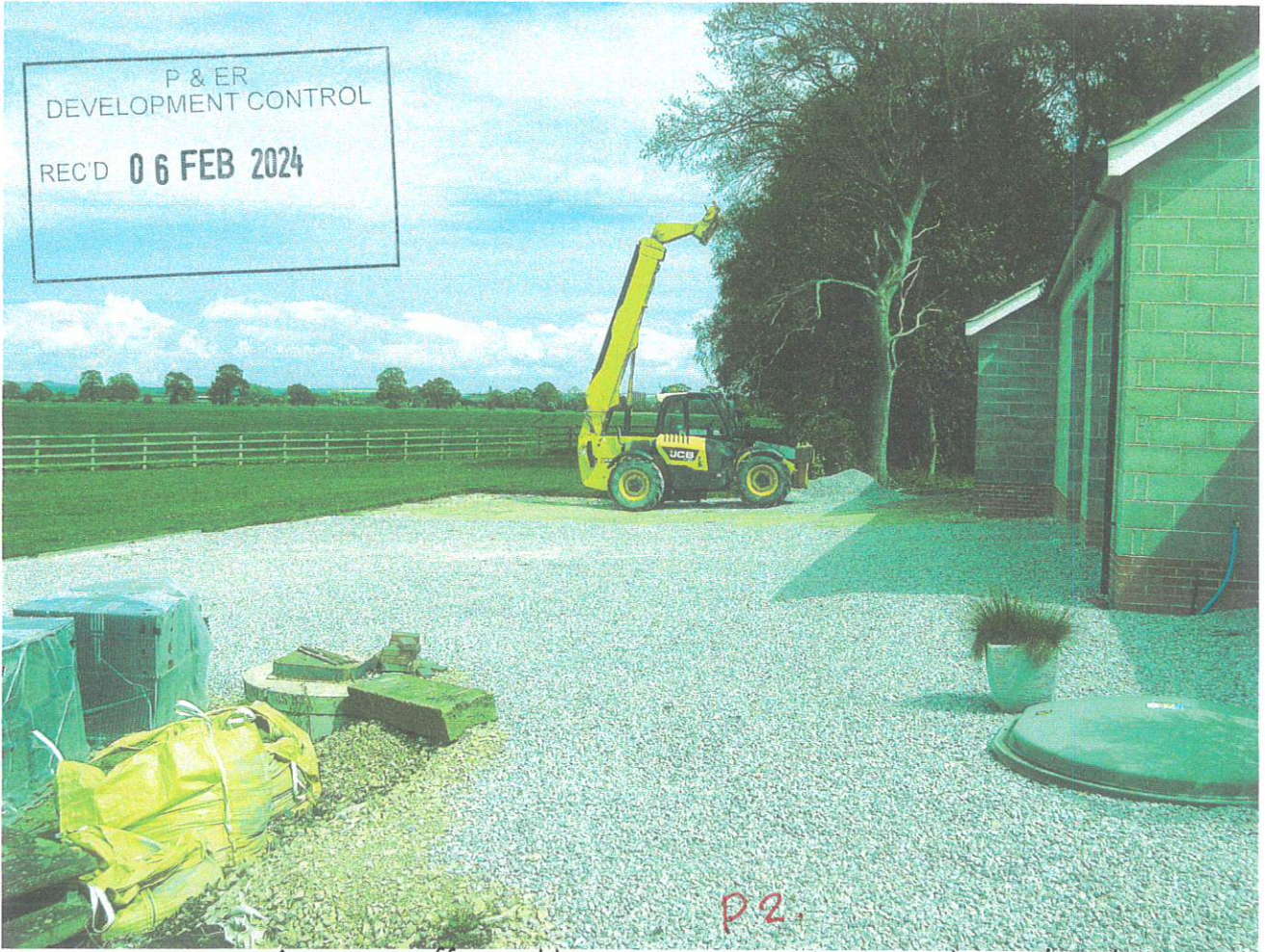
shows offloadin area and on site plant
