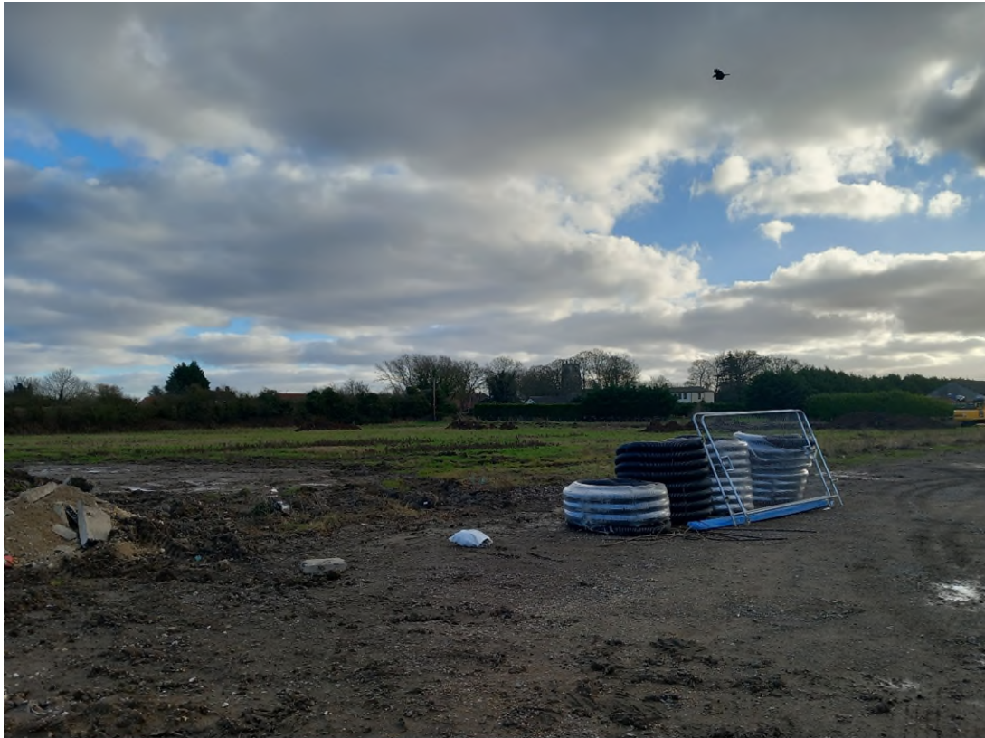
Plate 1 The development site as viewed from the north-west.
