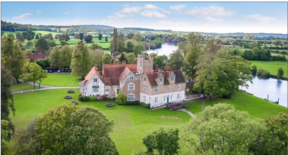
Images 4 & 5: Aerial Views of Bisham Abbey Site and Scheduled Monument.
