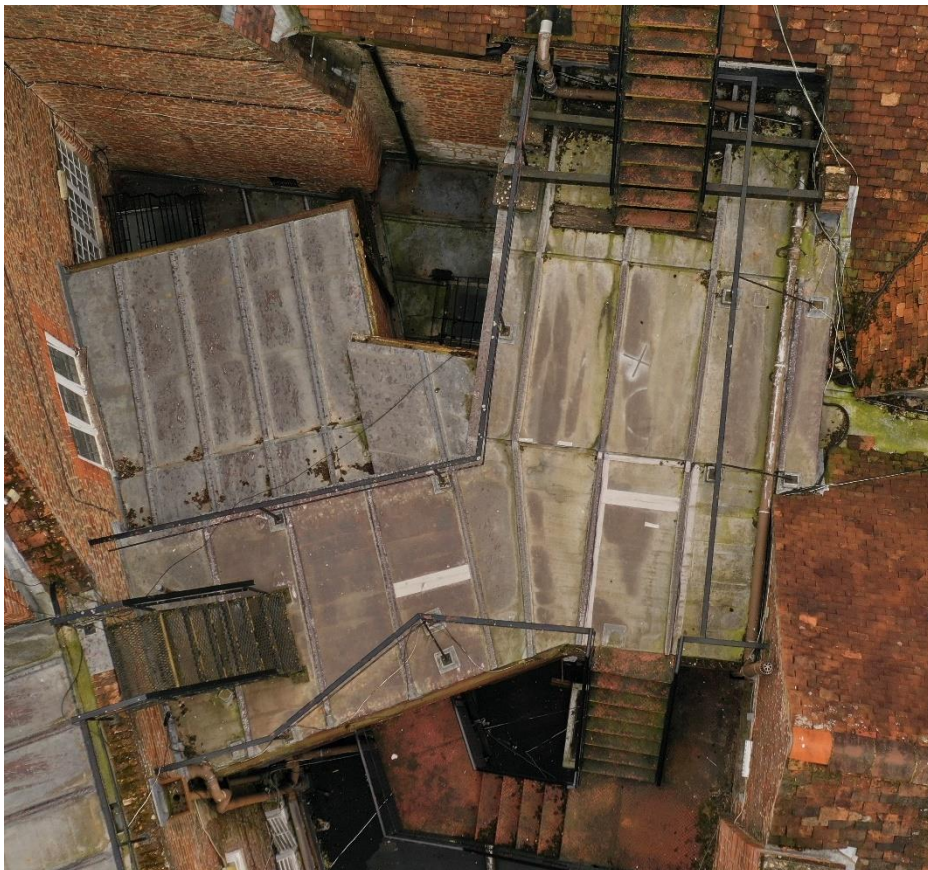
Roofs O1, O2 & O2 – Flat Lead
