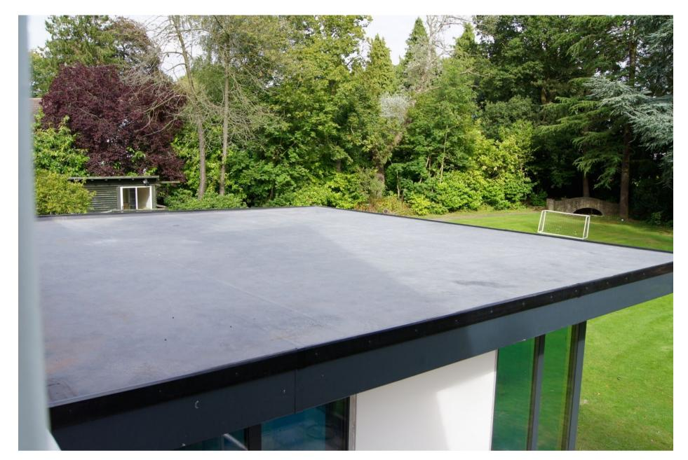
An EPDM rubber membrane will be used on the roof. The flat, sloping roof will have a low profile meaning the rubber membrane will only be visible from above.
