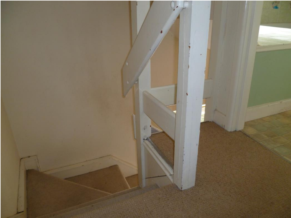
Photograph 2 – View looking down existing late 20 th century staircase from first to ground floor kitchen area and showing bathroom door to right.
