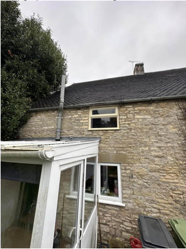
Photograph 3 – View showing rear elevation No. 13.
