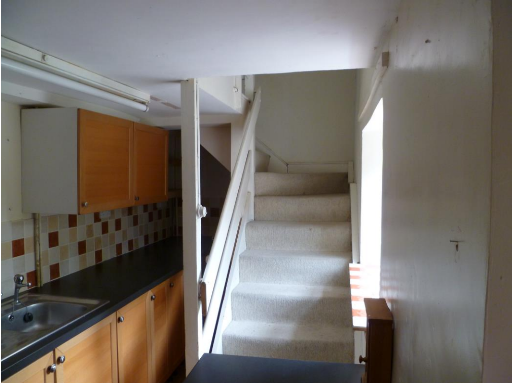
Photograph 1 – View looking towards late 20 th century staircase and showing the juxtaposition of kitchen units, lack of access to units and staircase discharging straight into kitchen units in the foreground.
