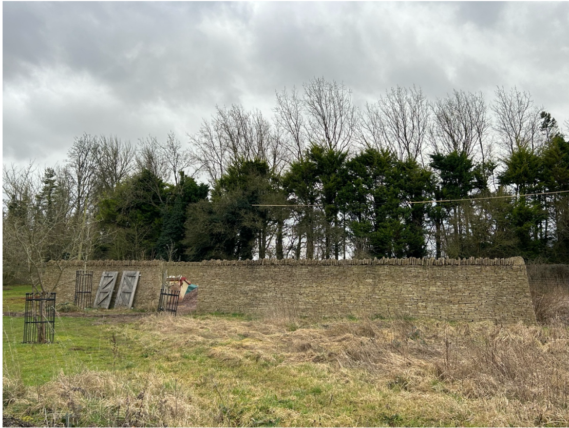
Image : Existing garden – as viewed from the north
