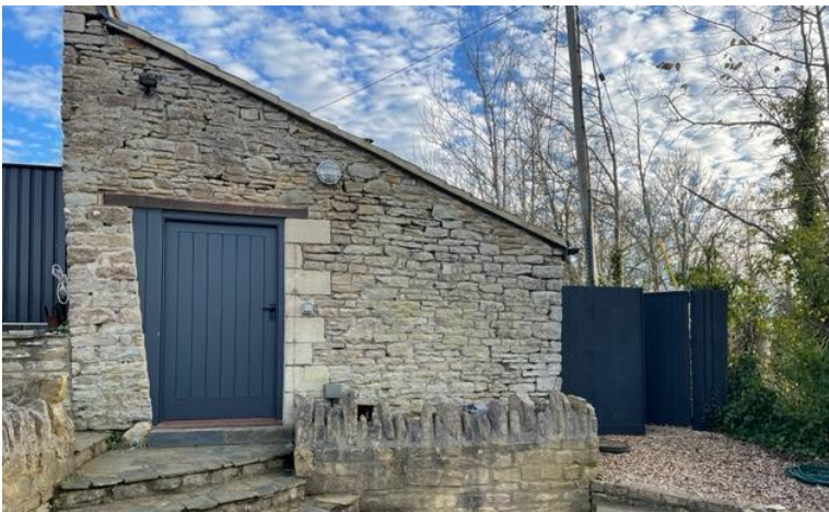
The north-west elevation is unchanged when viewed from the main house.
