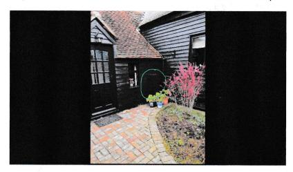
Photograph with augmented reality, imposed Hypervolt car charger in proposed position. Green drawn line shows where black cable will be 'run' from external meter box
