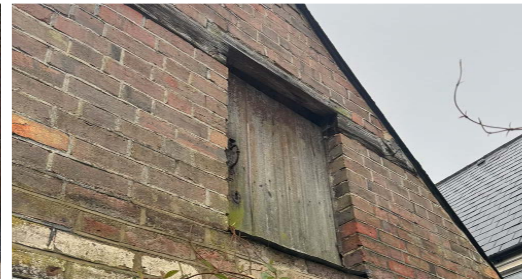
Figure 4.0 - Current Access at rear garden from Albert Street & Akeman & original features.
