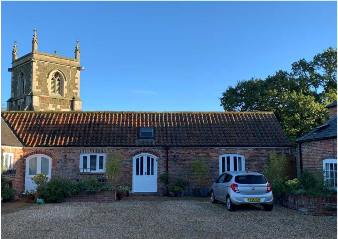
Figure 2: Location from South Elevation
