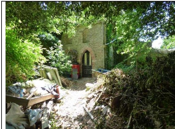
Photo 4: Waste materials beside the structure (TN2 of Figure 2).
