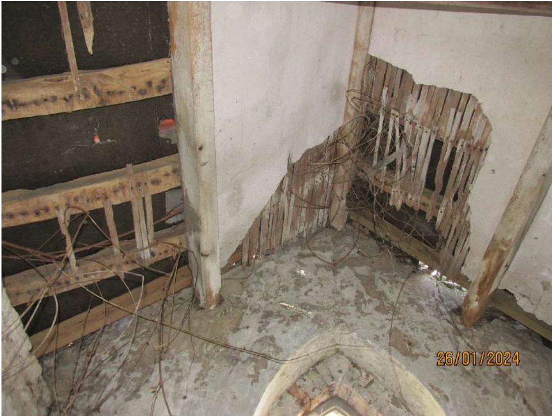
Internal Elevation of west gable wall showing roof structure
