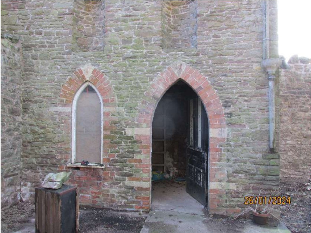
External north elevation of building – Ground Floor
