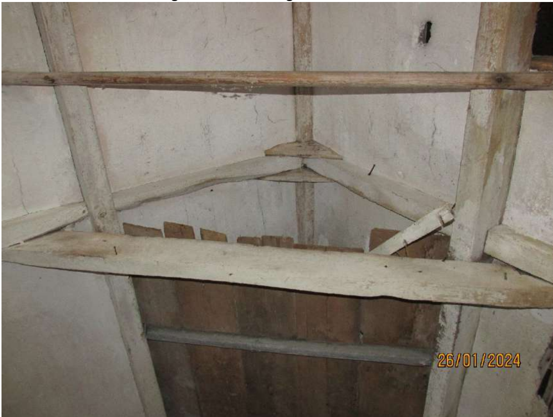
Internal Elevation of roof showing rudimentary truss
