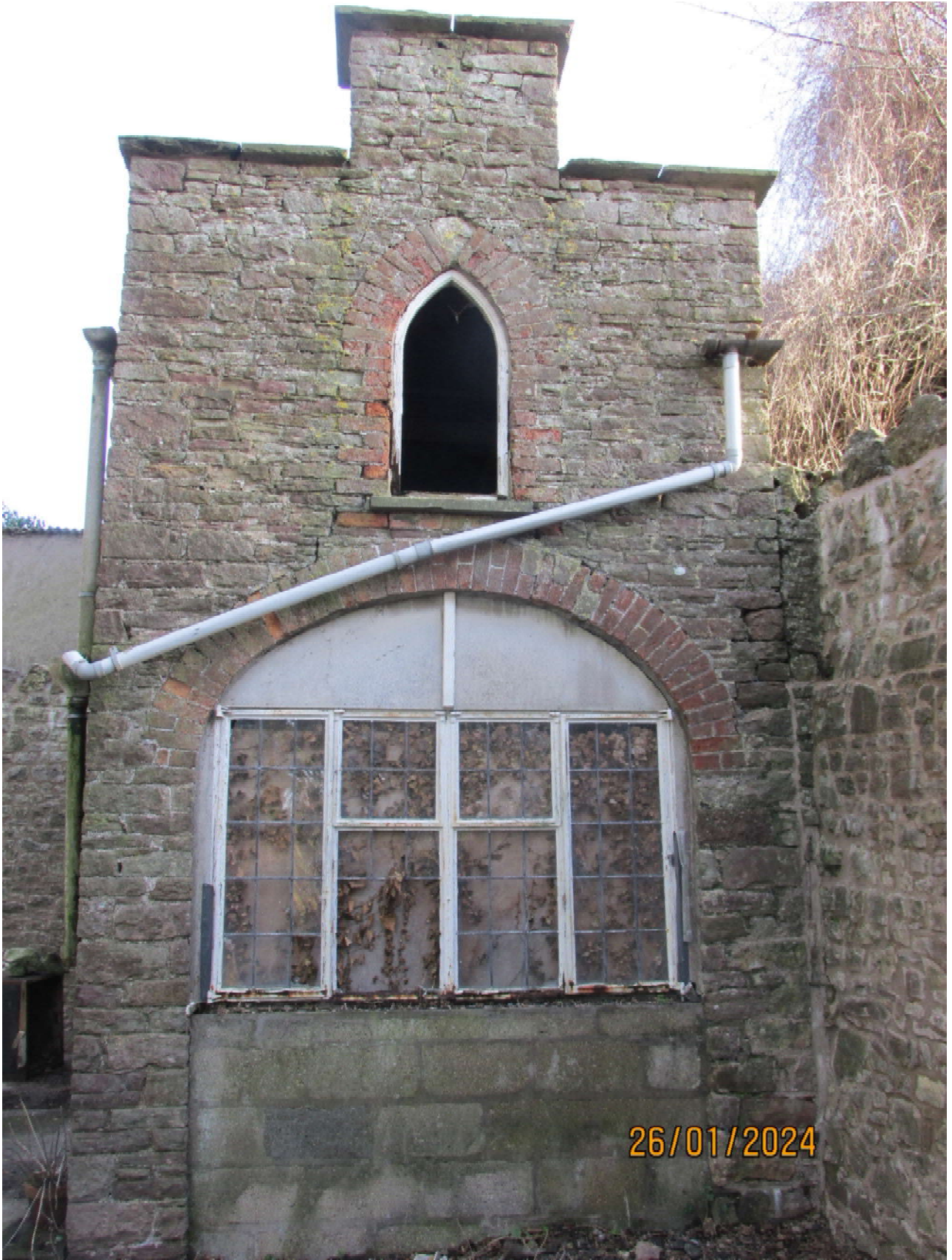
External west elevation of building
