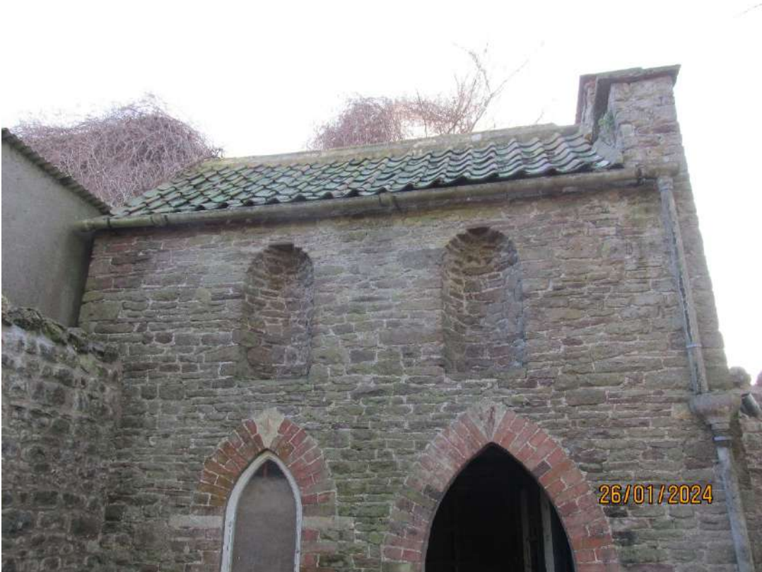
External north elevation of building – First Floor
