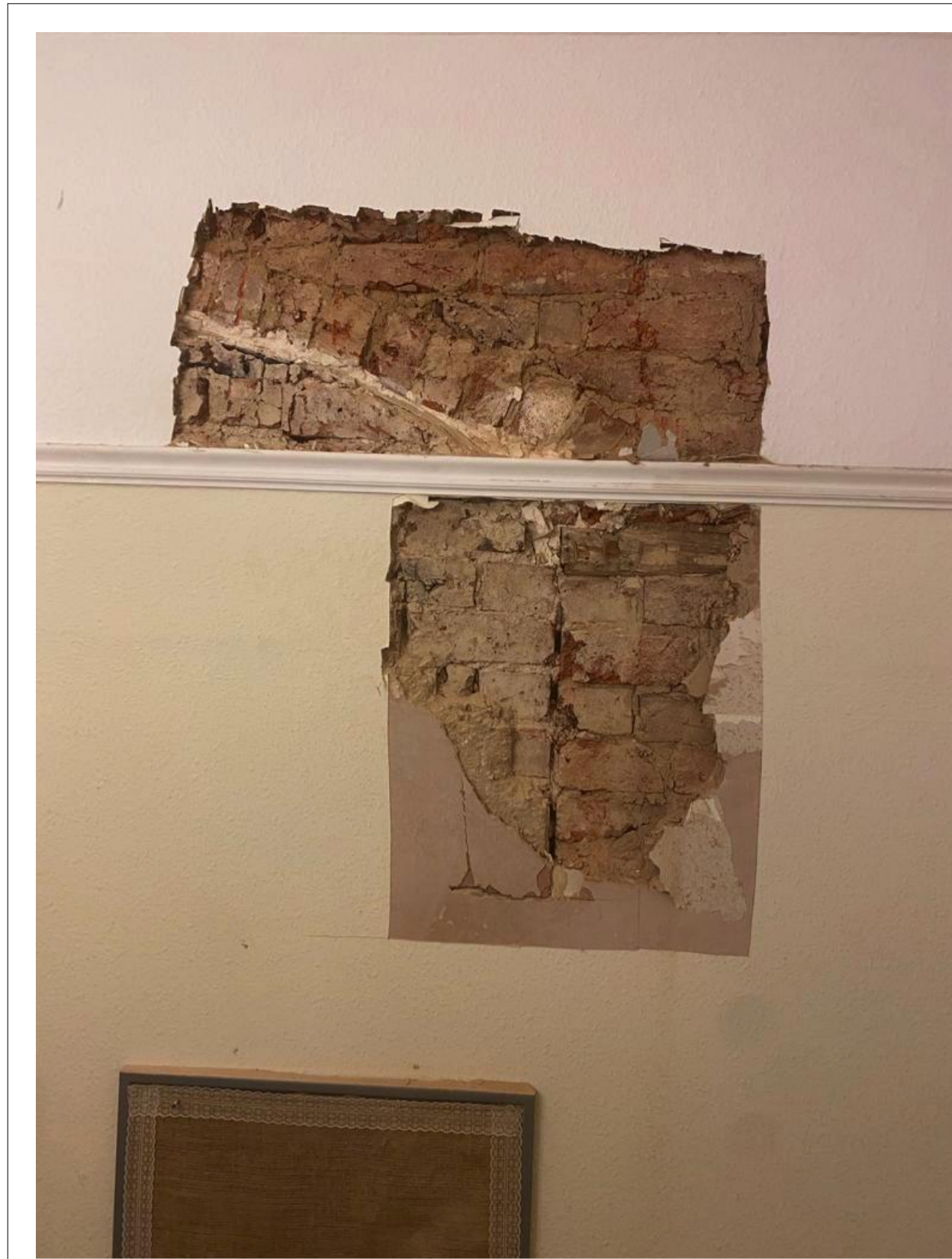
Existing Archway revealed behind plaster
