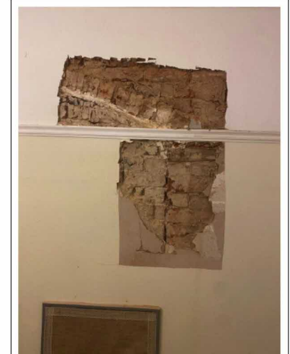
Existing Archway revealed behind plaster
