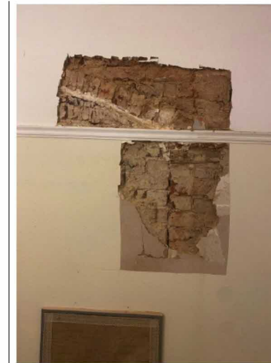
Existing Archway revealed behind plaster
