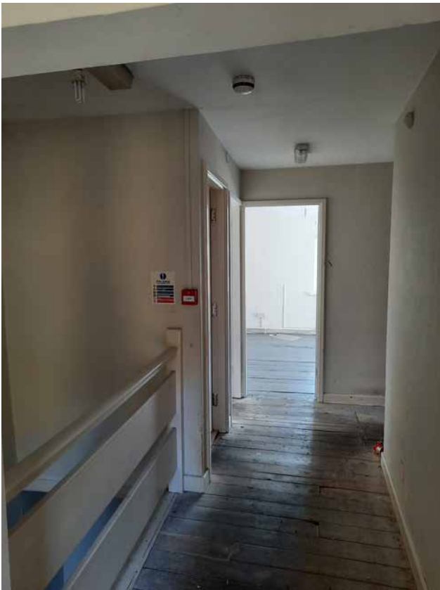
3.44a Central corridor at first floor with modern stud partitions
