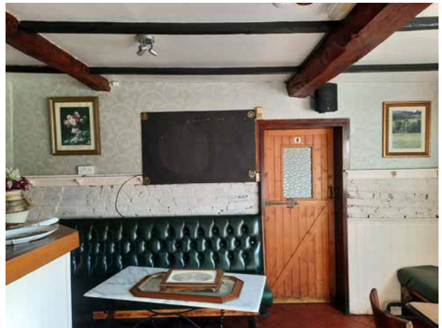
3.40 Timber beams and access to WCs in altered stores
