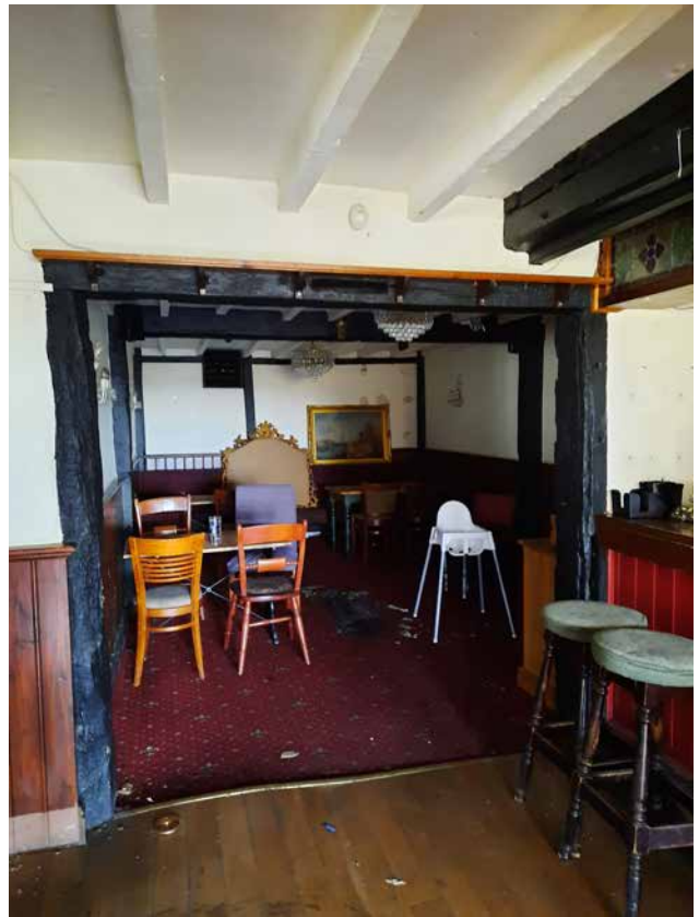
3.39 Original timbers at ground floor
