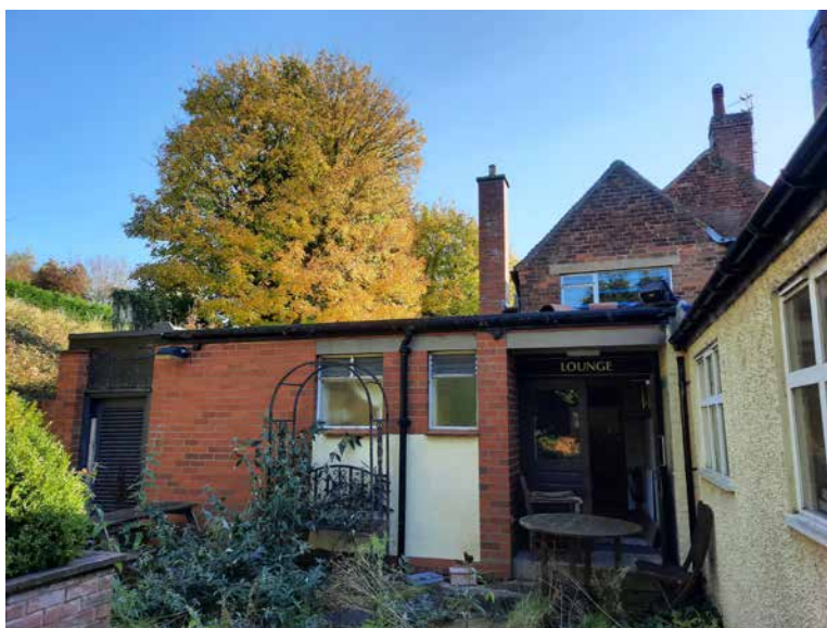
3.33a Side (west) elevation with build up of detracting extensions
