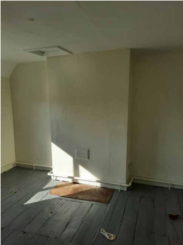
3.46a Original chimney breast to west of first floor
