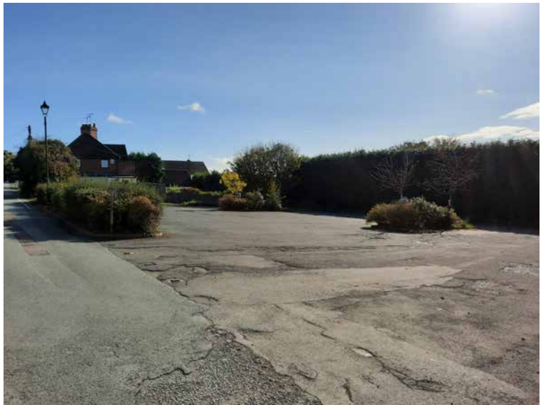
3.47a Carpark site facing
