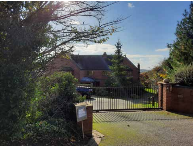
3.8b Pennwood Lane - Pennwood House
