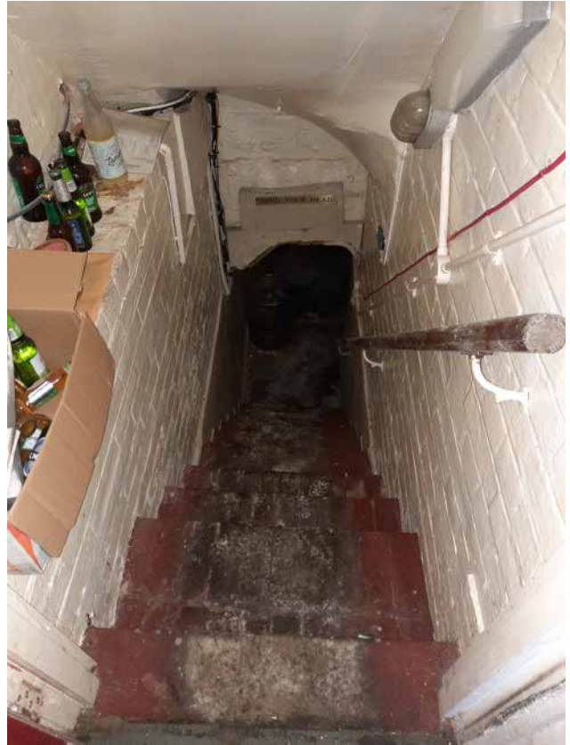
3.35b Brick stairs down to cellar
