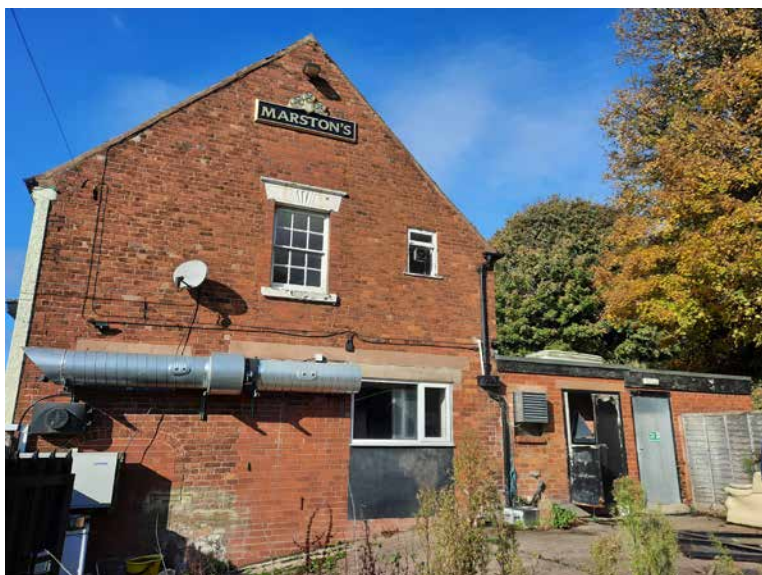
3.32 Side (east elevation) with build up of detracting alterations and additions
