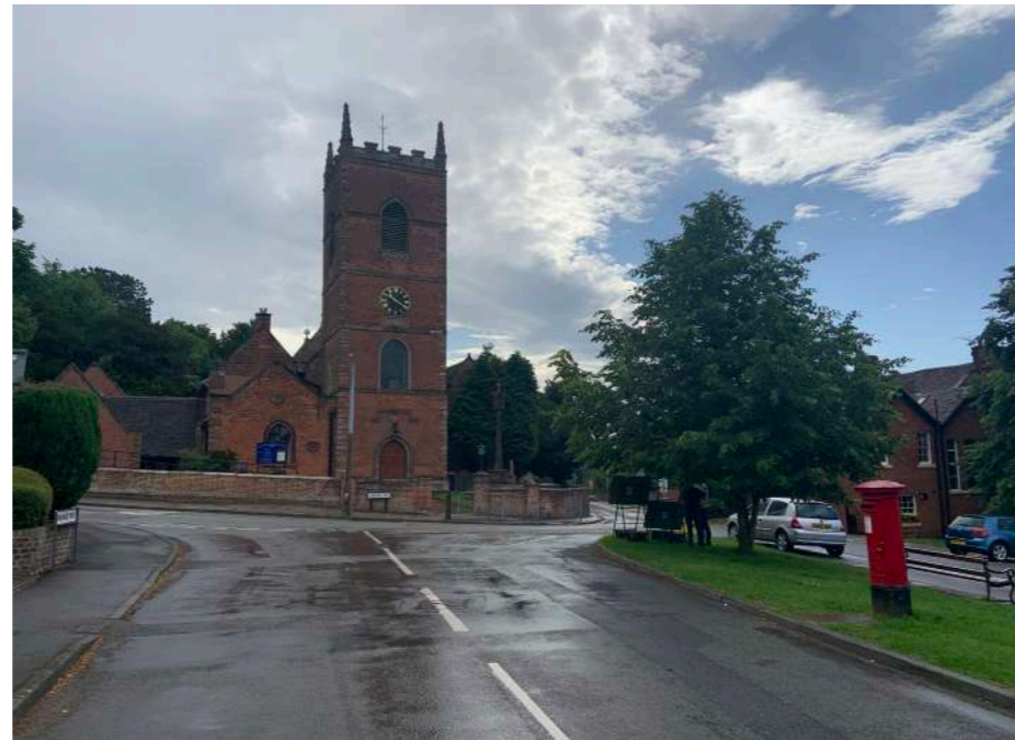
2.3.3.2 View 9 - Front elevation of Grade II* listed St Bartholomew's Church
