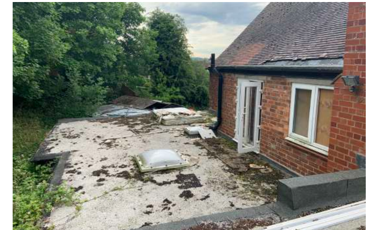
2.5.3 Poor quality single storey extensions to rear of pub
