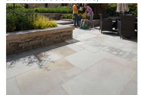
3.7.5 Stone paviors to patio area
