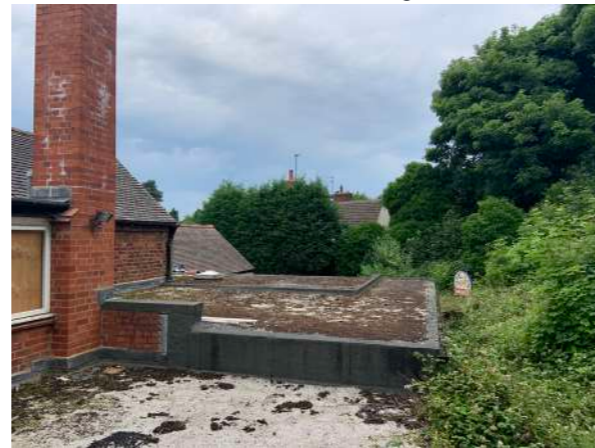
2.2.4 View west from roof of rear extension
