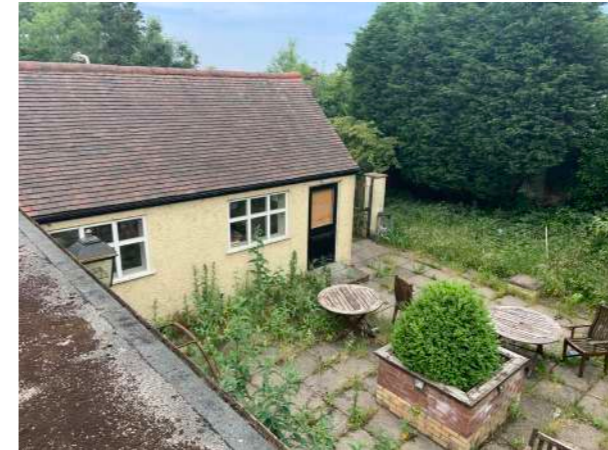
2.2.2 Former outdoor seating area to the west
