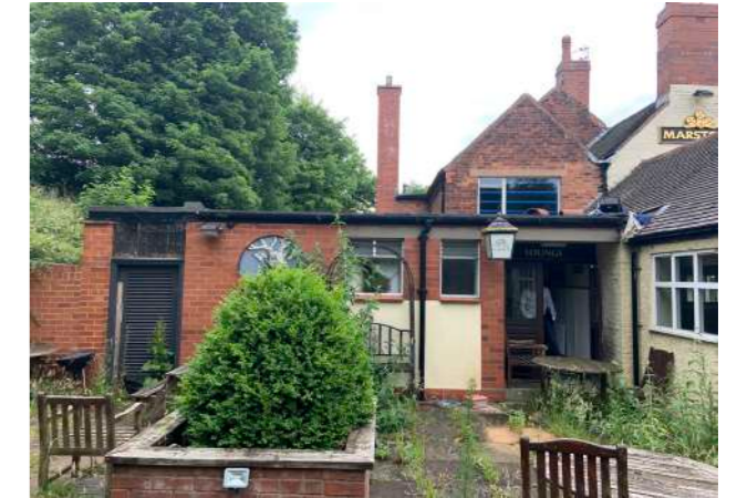
2.2.3 View from outdoor seating area towards rear extension
