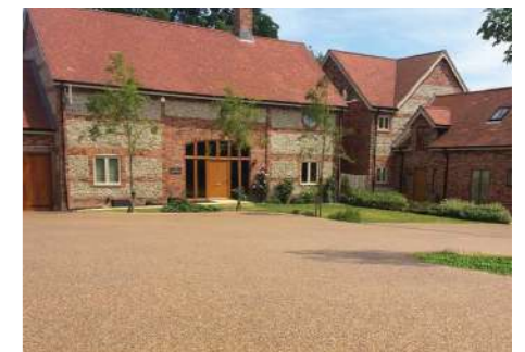
3.7.4 Resin Bound Gravel Driveway
