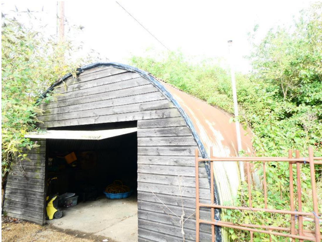
Photo 11 , east and south aspects of building three, looking northwest.
