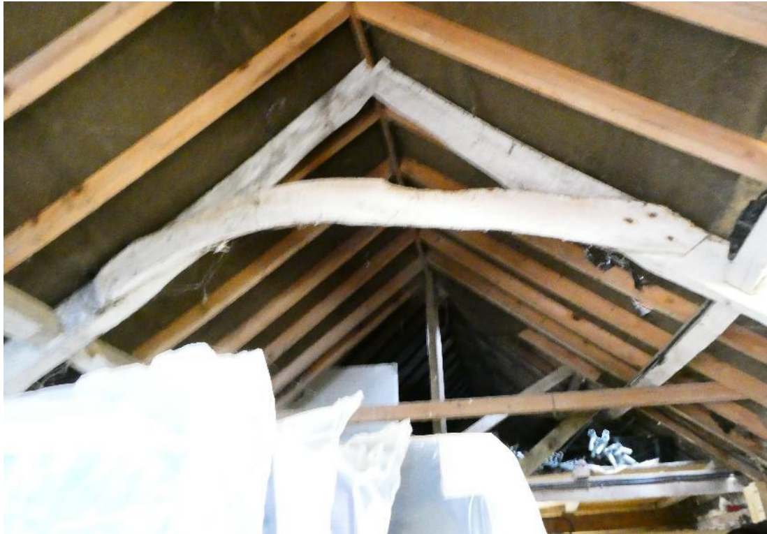
Photo 6 , internal view of building one, looking north.
