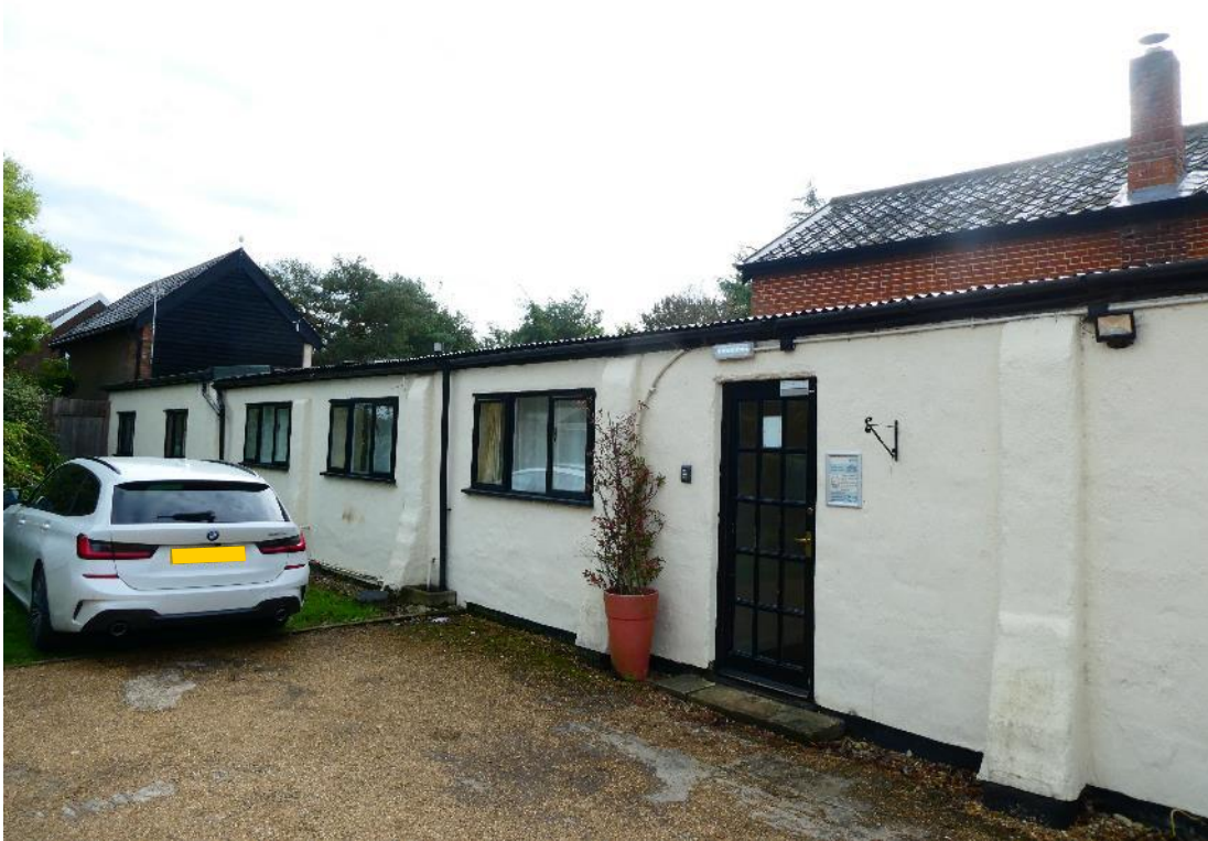
Photo 7 , north aspect of section A, looking southeast.
