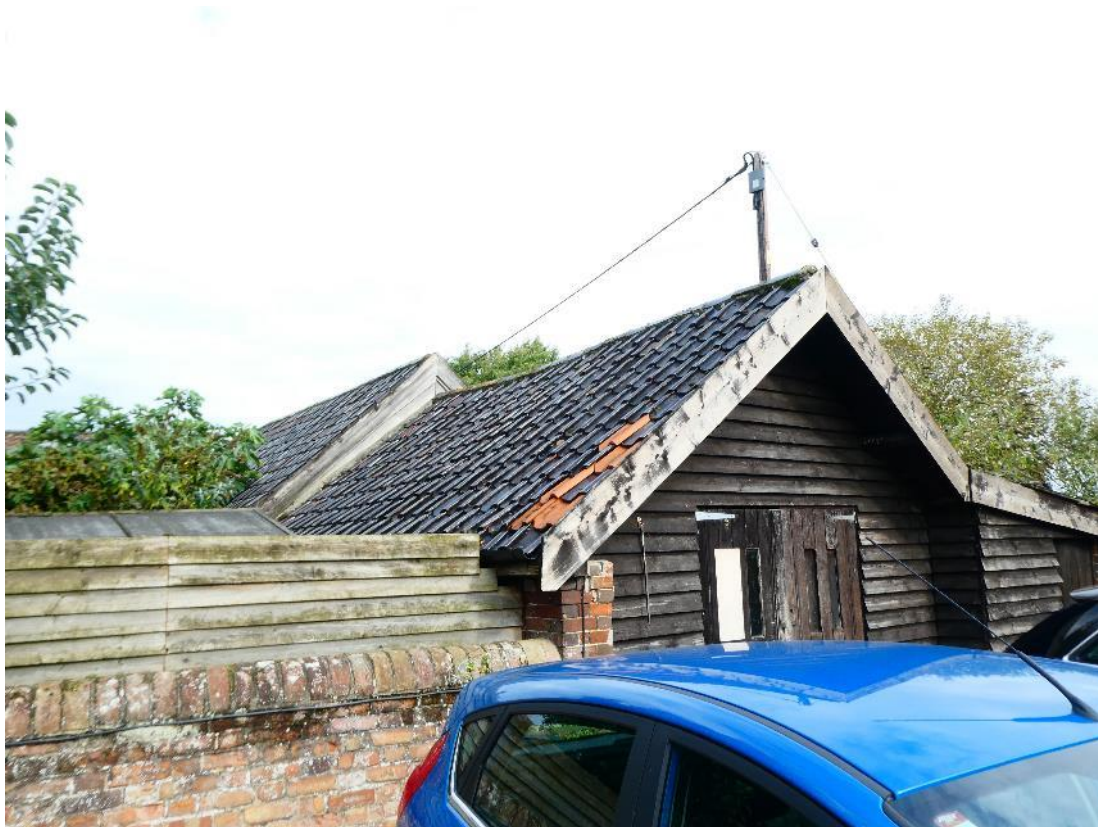
Photo 3 , south and west aspects of building one, northeast.
