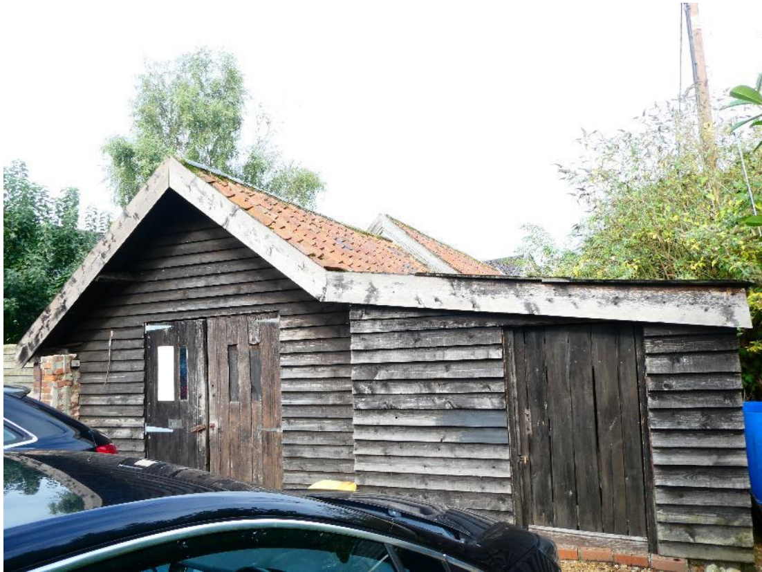
Photo 4, east and south aspects of building one, looking northwest.
