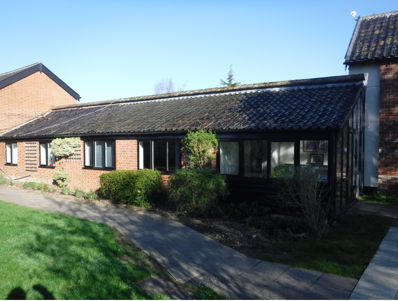
Phase II existing modern extension pantile roof:
