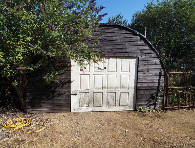
Phase I Lean-to to be demolished:
