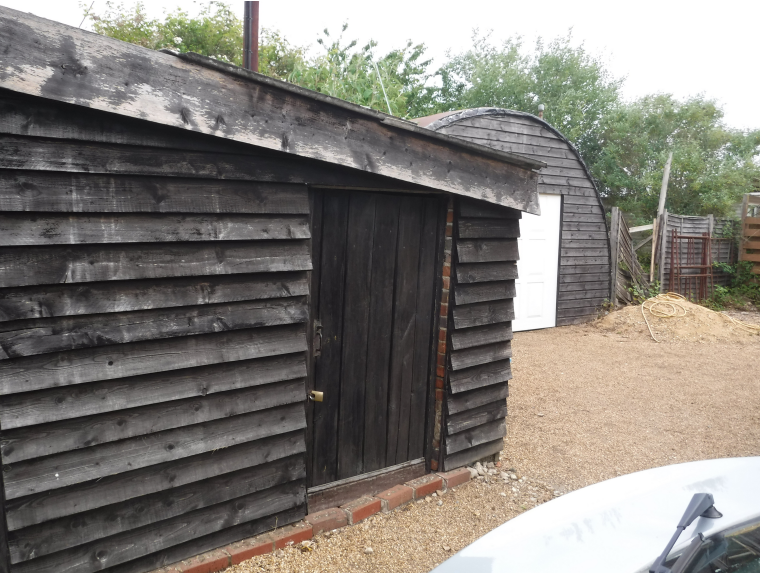
Phase II existing roof mixed construction:
