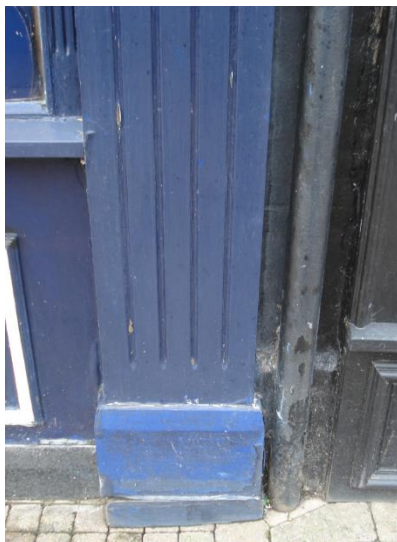
Existing timber shopfront showing dilapidated panels.
