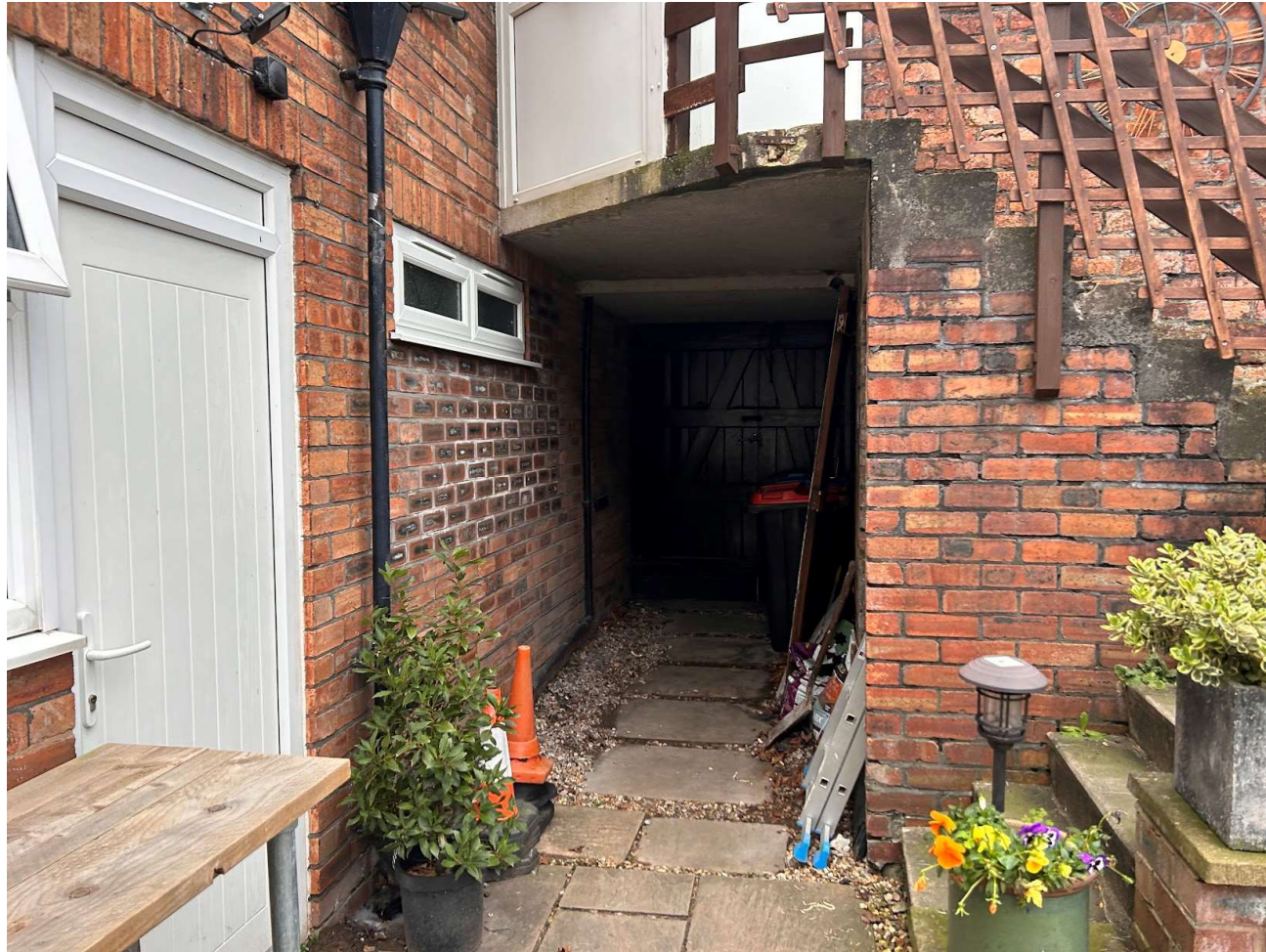
View of existing rear covered passage
