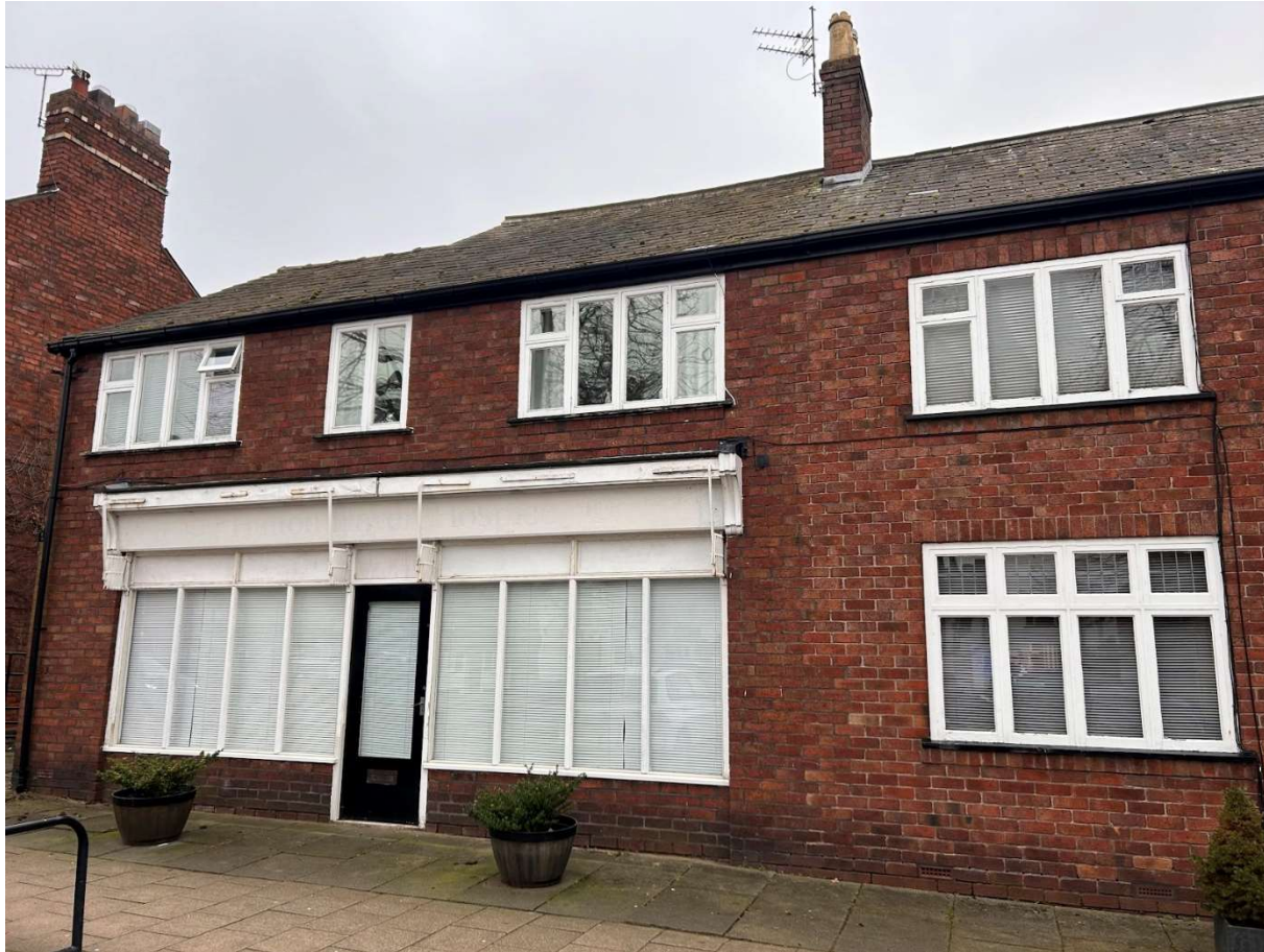
Existing front elevation, showing existing shop front
