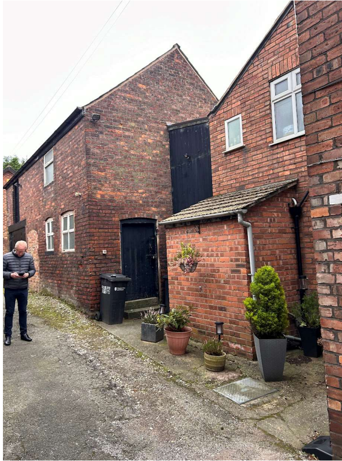
Existing view Southwards from side of property along vehicaulr access of existing small lean-to, proposed to be carefully removed.
