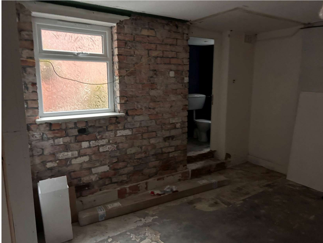
Internal view of existing shop rear area
