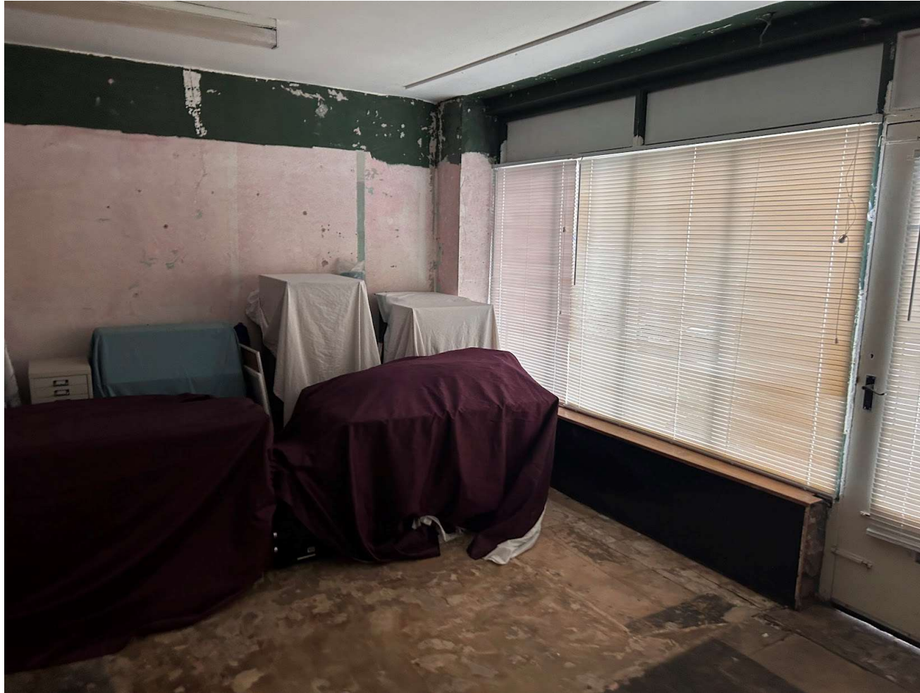
Internal view of existing shop front area
