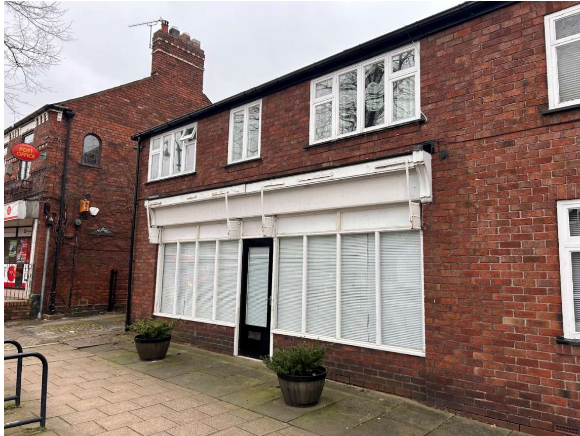
Existing front elevation, showing existing shop front
