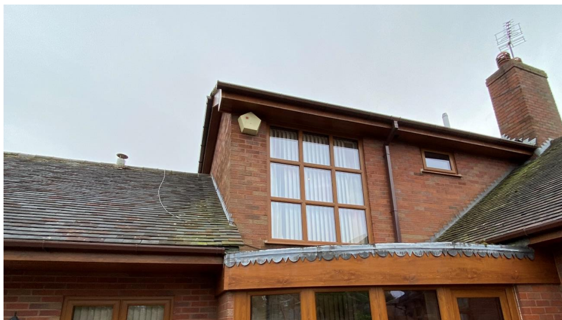
Fig. 1. Showing modern brickwork at first floor level
