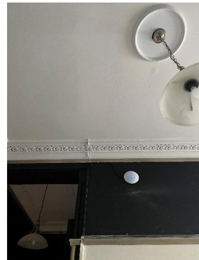
Stairwell embedded wiring and light fitting
