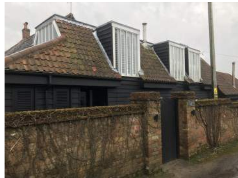
Existing pedestrian gate on road elevation. To be retained
