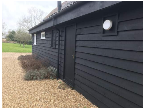
Existing doorway to be adapted for new boot room entrance
