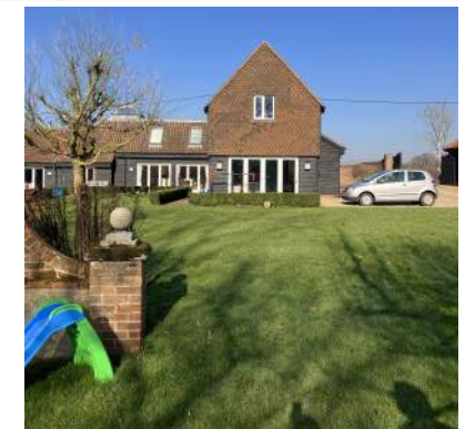
View towards rear of house showing topography falling away from house
