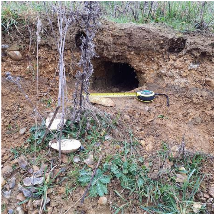
Photo 22. Burrow in the SW side of the pond H excavation.
