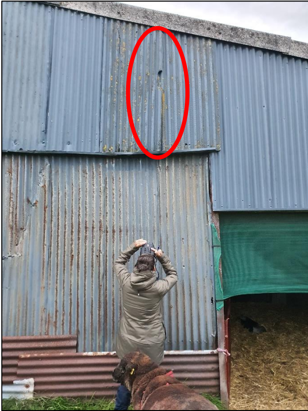
Plate 6: View of southern elevation of the large barn showing the location of the identified maternity, colonial roost site for an observed ten common pipistrelle bats
