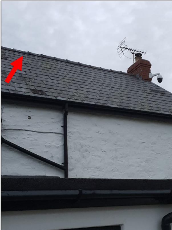
Plate 3: View of the S roof slope of the main (southern) part of the house showing location of solitary common pipistrelle bat roost at the ridge
