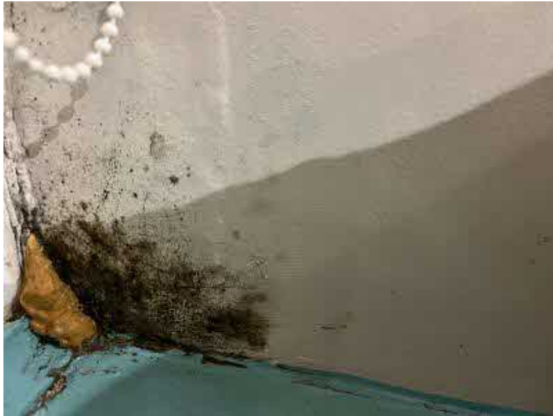
living room ceiling
