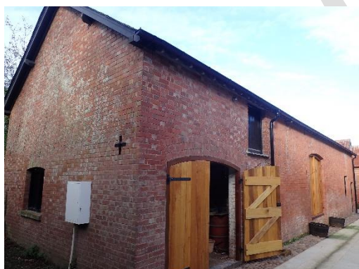
Figure 2. The south and east elevations of Barn C
