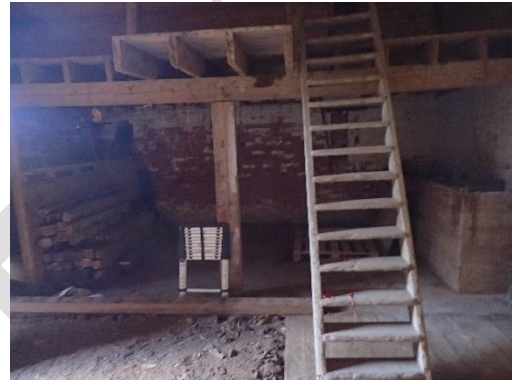
Figure 9. The central section mezzanine floor
