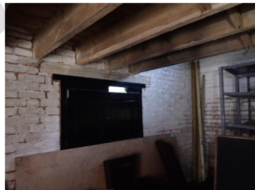
Figure 15. Free-flight access via louvered opening in south gable ground floor window
