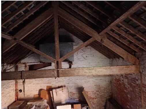
Figure 8. The central section viewed from the mezzanine floor
