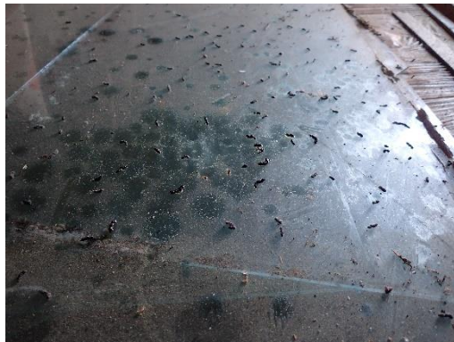
Figure 12. Mixed droppings and urine staining on stored items within the barn
