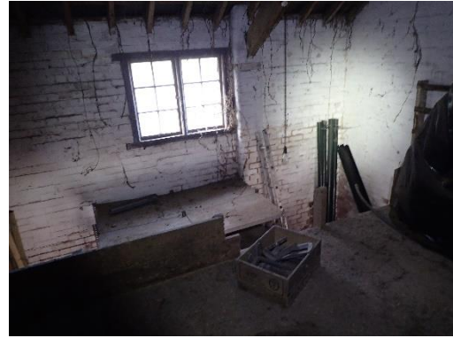
Figure 7. The south section mezzanine floor
