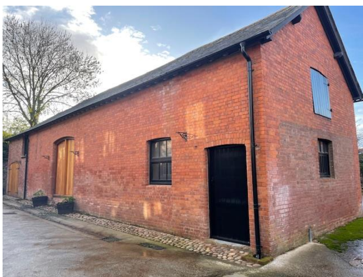
View of the Existing Barn
