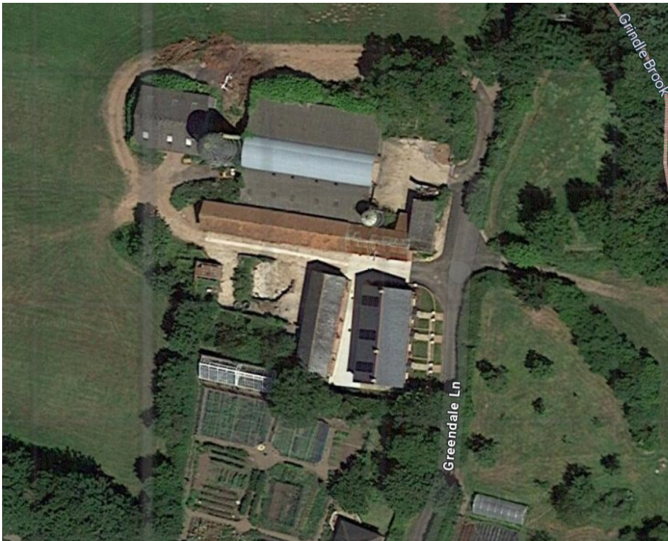
Fig 5. Google Earth Extract 2023: Greendale Farmstead
