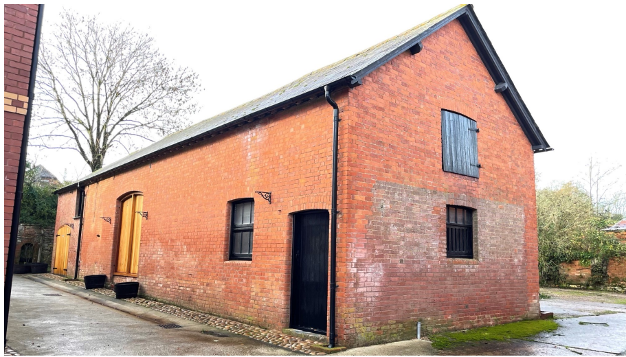
Fig 8. Existing Photo; Barn C (East & North Elevation)
