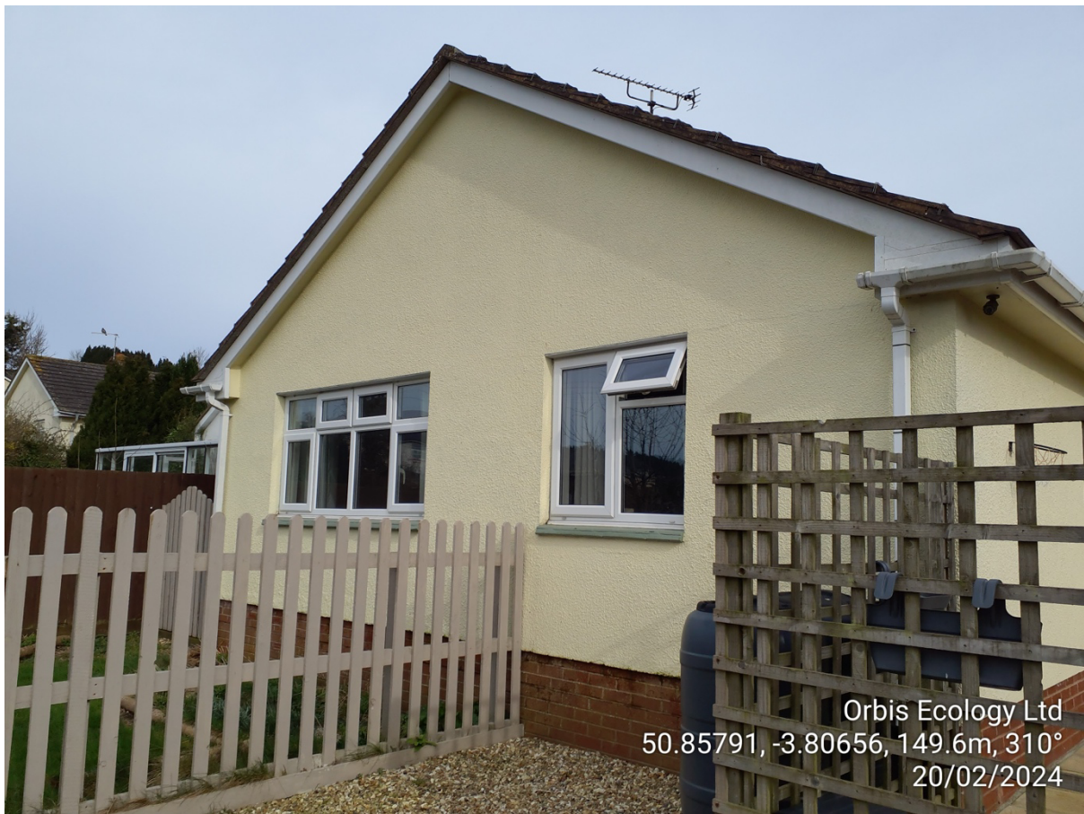
Rear of the property to be extended
