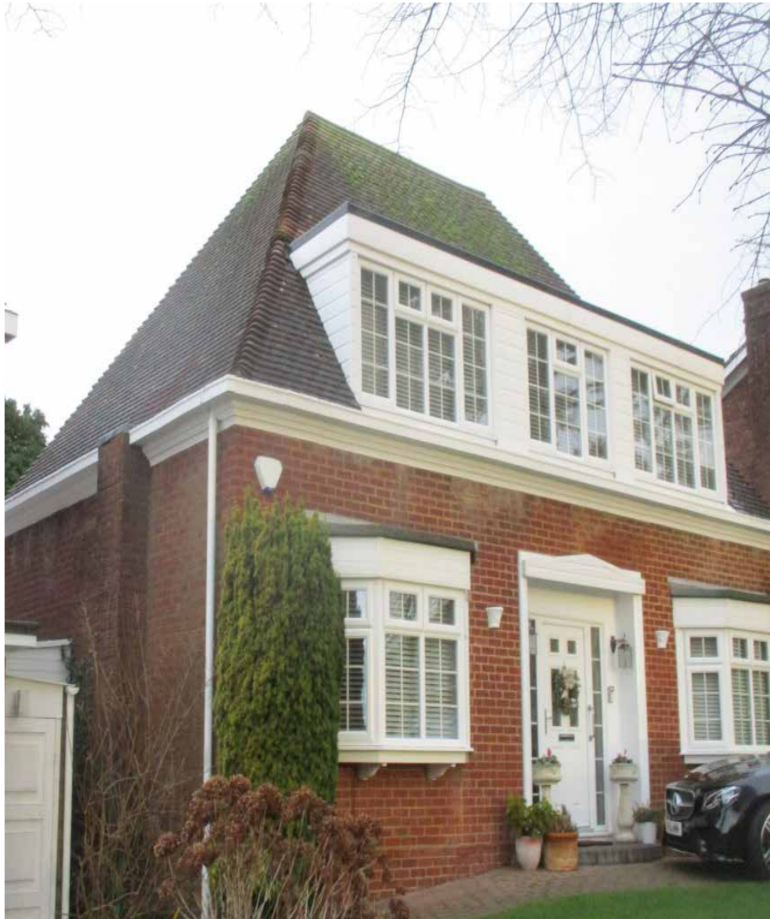
Fig. 4: Front elevation of existing house.
