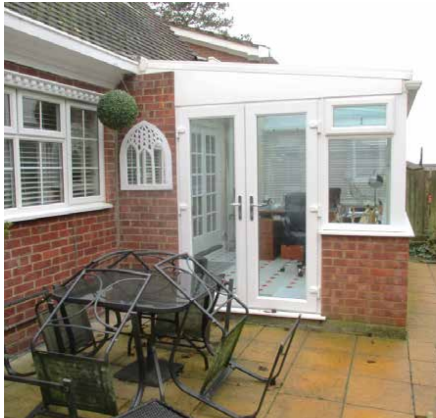
Fig. 9: Rear view showing existing conservatory
