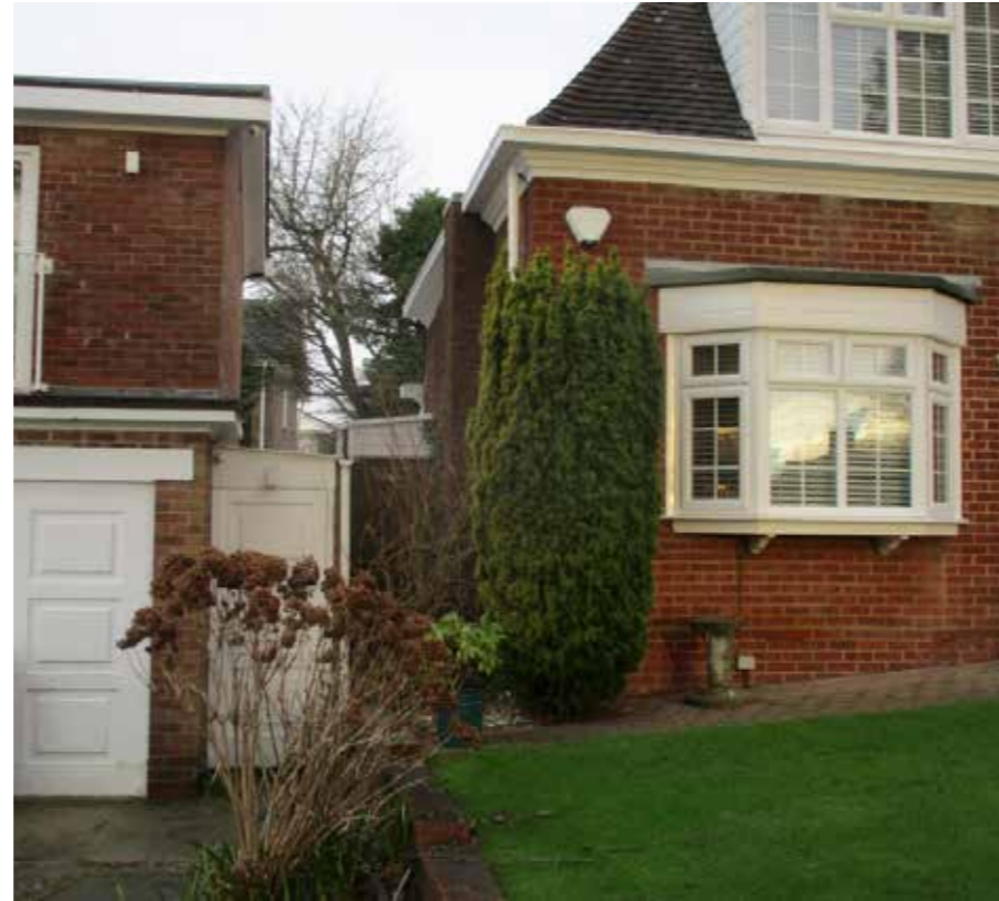
Fig. 7: Front view of existing side store to be removed
