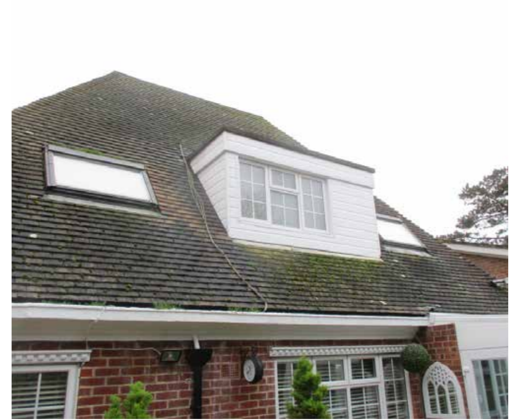
Fig. 11: View of existing roof light to be replaced and existing dormer to be retained with amendments
