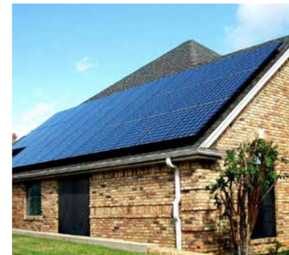
Sustainability Technologies - Solar Panels
