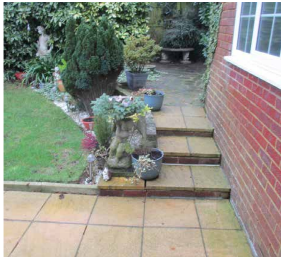
Fig. 10: View of rear hard landscaping to be removed
