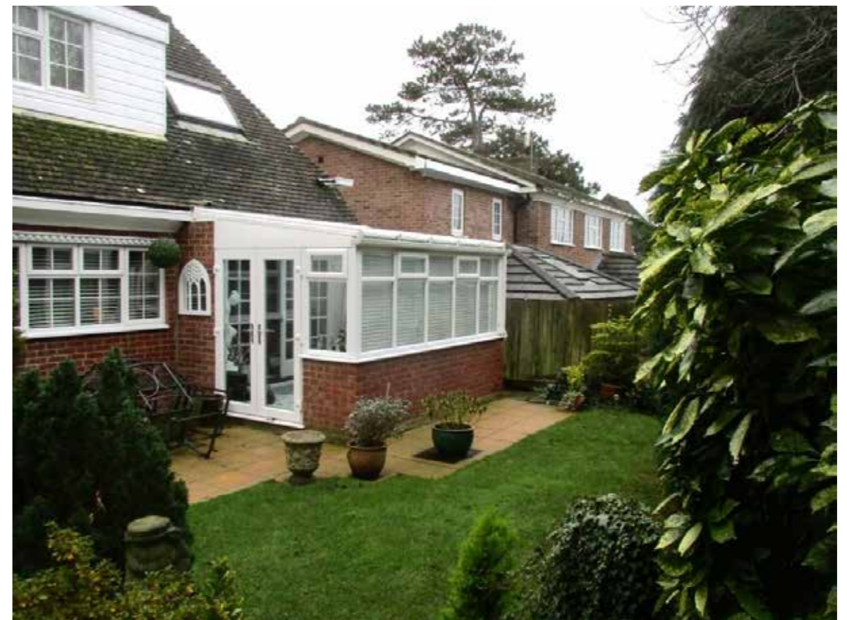
Fig. 5: Rear elevations of existing house
