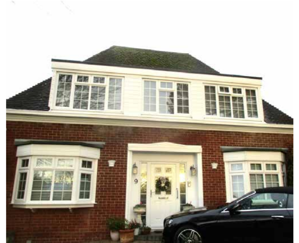
Fig. 8: View of the existing fenestrations to be retained
