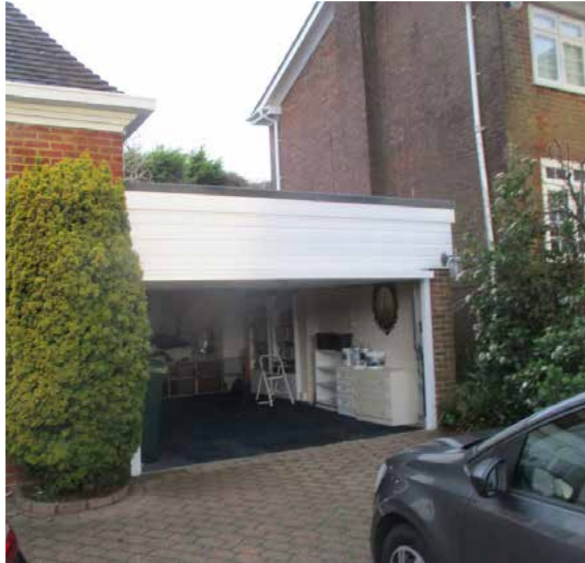
Fig. 6: Front view of the existing garage proposed to be refurbished
