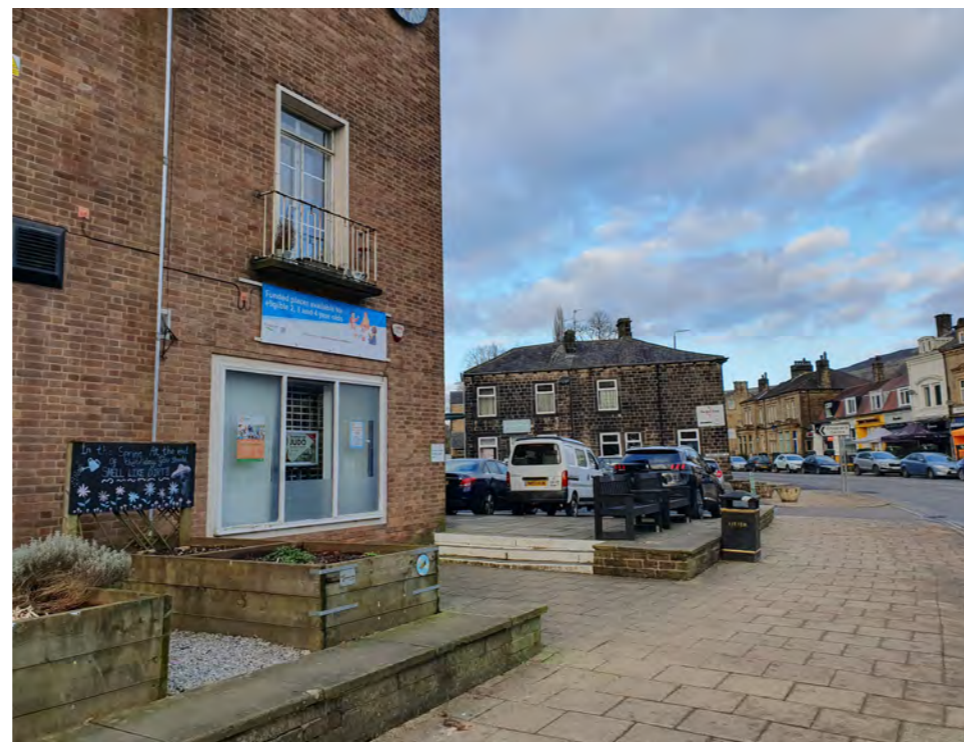
View of A646 street frontage including steps and planters
