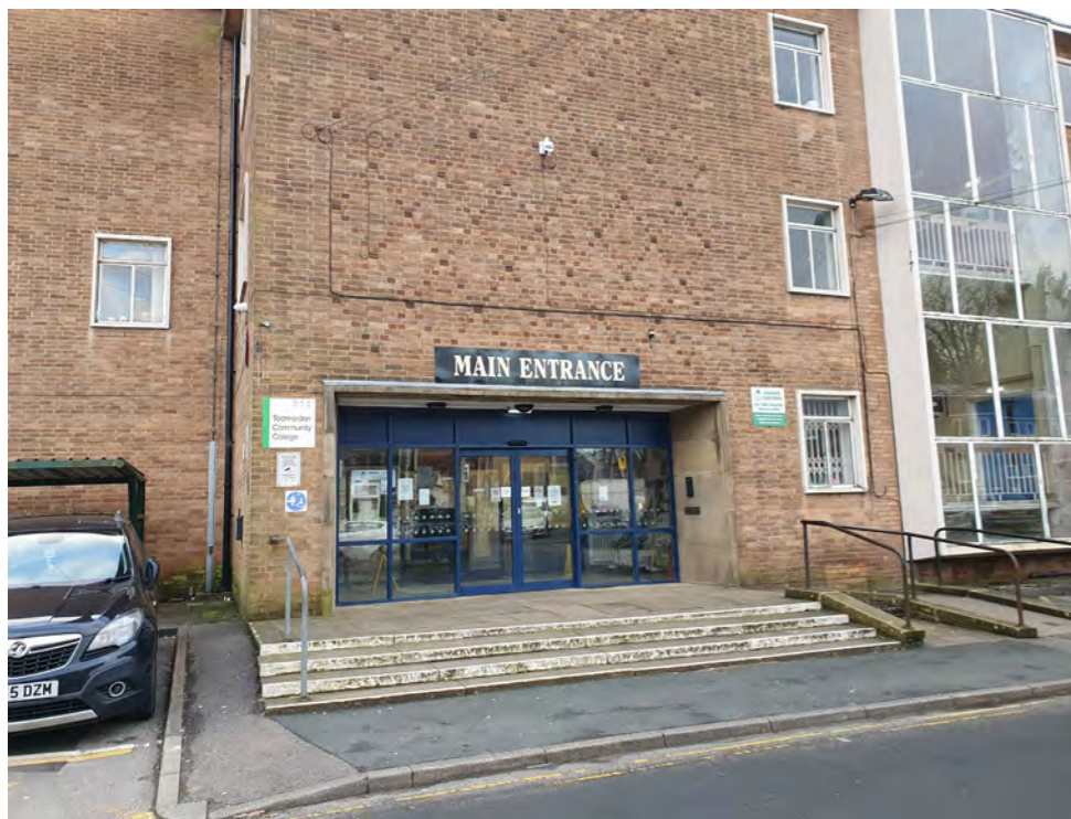
View of main entrance, steps and ramp
