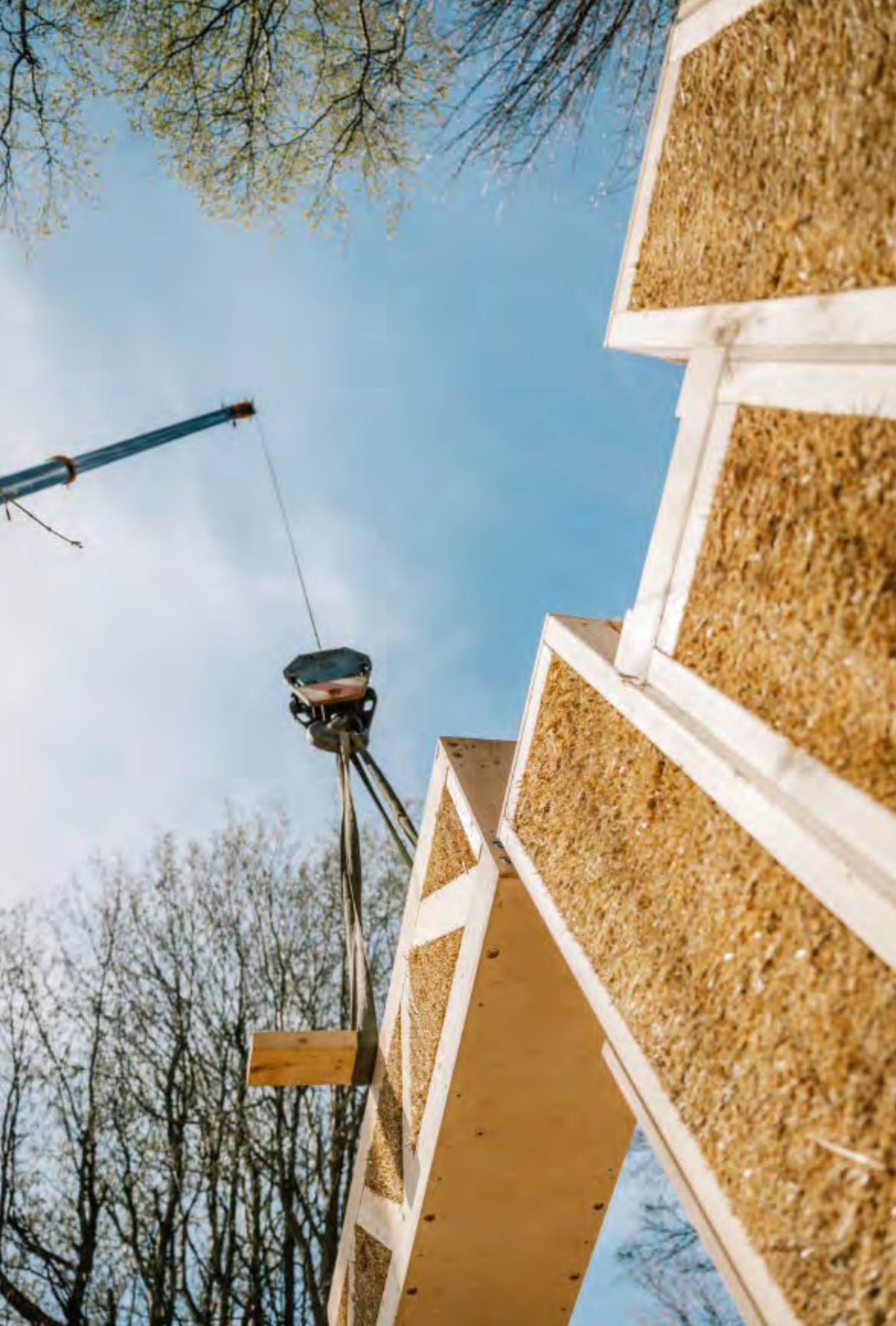
Straw insulation panels being installed
