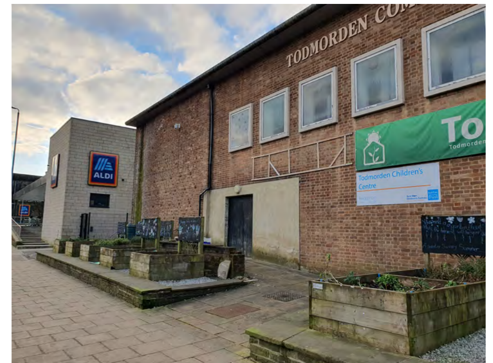
View of raised planters and fire exit onto A646 street frontage
