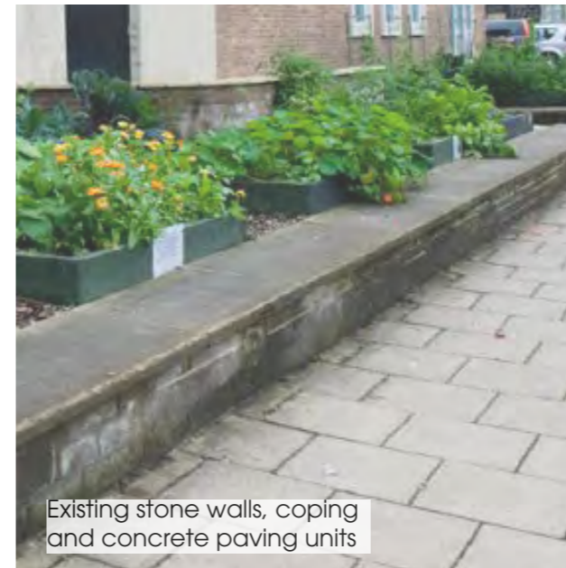
Wall made from re-purposed concrete paving units
