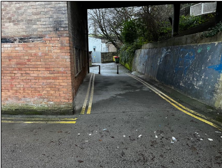
View of southern elevation showing the basement light well with a cast iron grill cover
