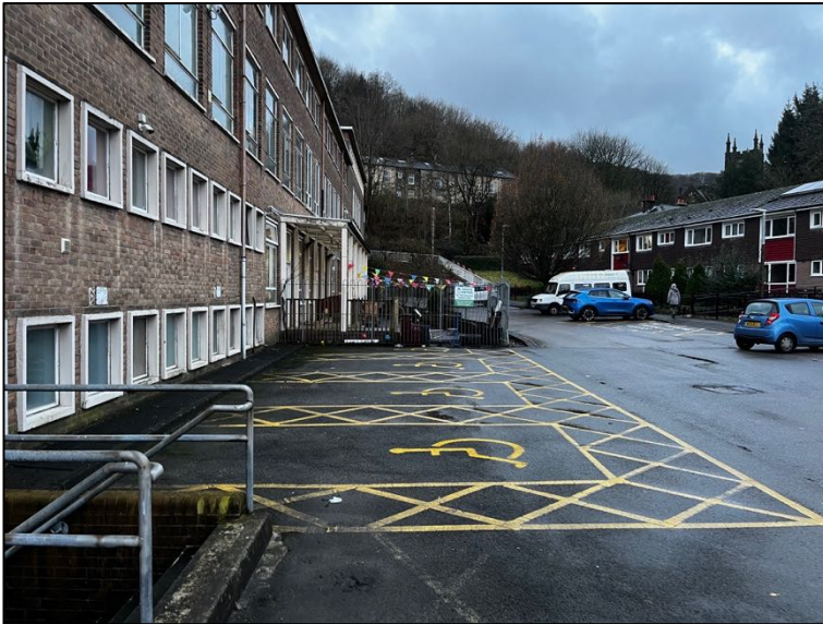
General view to the west along north elevation of the building and car park
