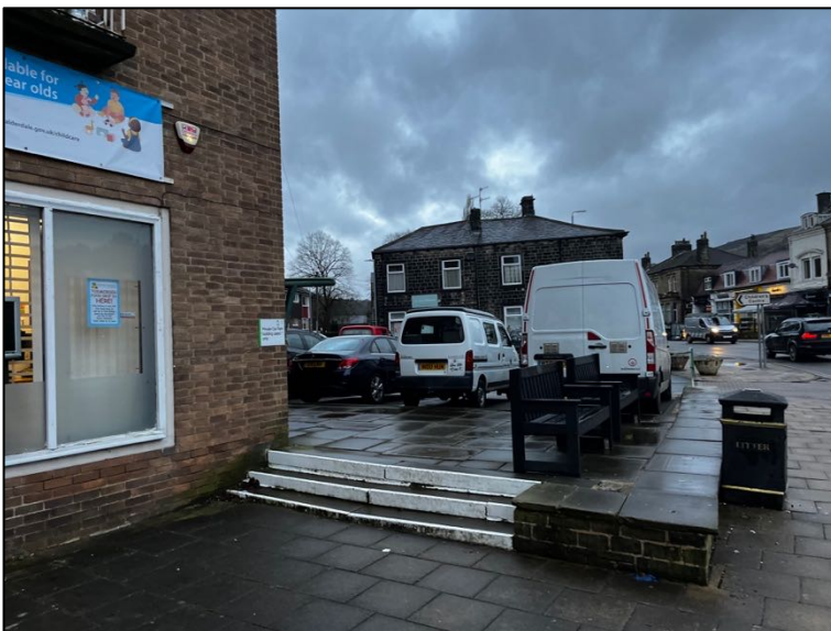
View of new flood protection adjacent to the River C
