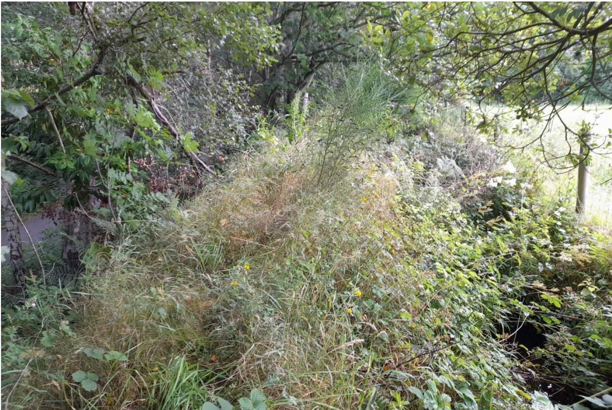
Figure 2.6 View looking east from the siphon outlet. The channel is visible in the bottom right, and is elevated above the Deeside Way footpath visible on the left.
