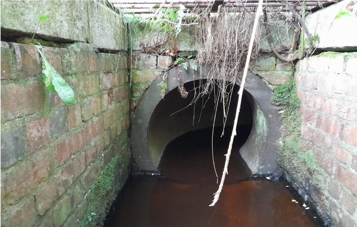
Figure 2.5 View looking upstream at the outlet face of the siphon which carries the watercourse beneath the Deeside Way footpath
