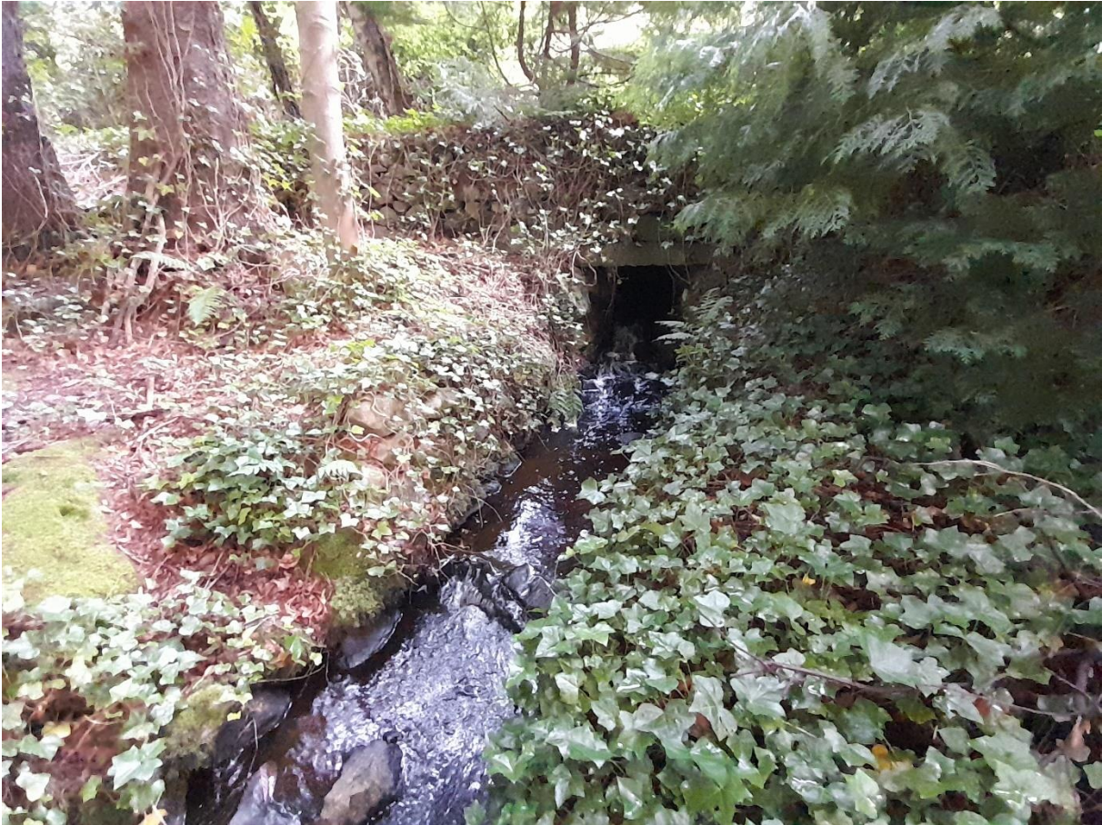
Figure 2.4 View looking upstream at the downstream outlet of the culvert passing beneath North Deeside Road.
