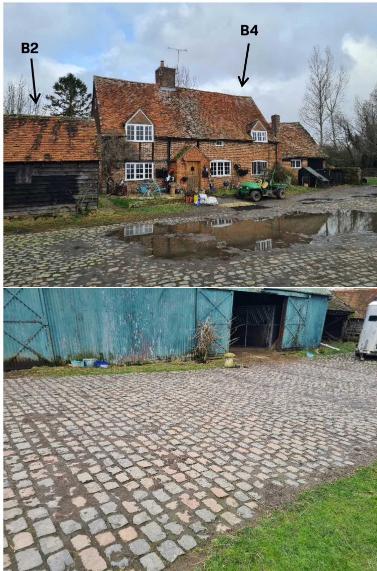
Figure 1: View from the stable yard, looking north at the dwelling (B4) and corner of the timber-framed barn (B2).
