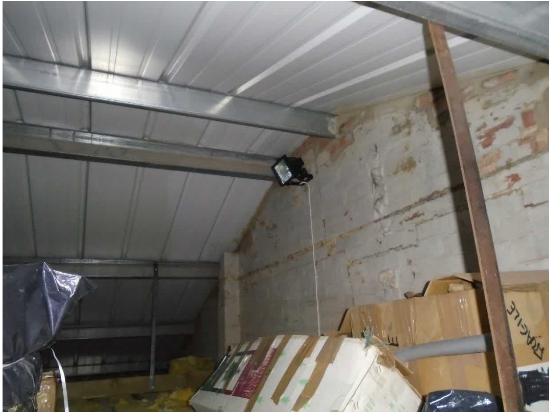
Rendered / sealed attic space with no bat evidence
