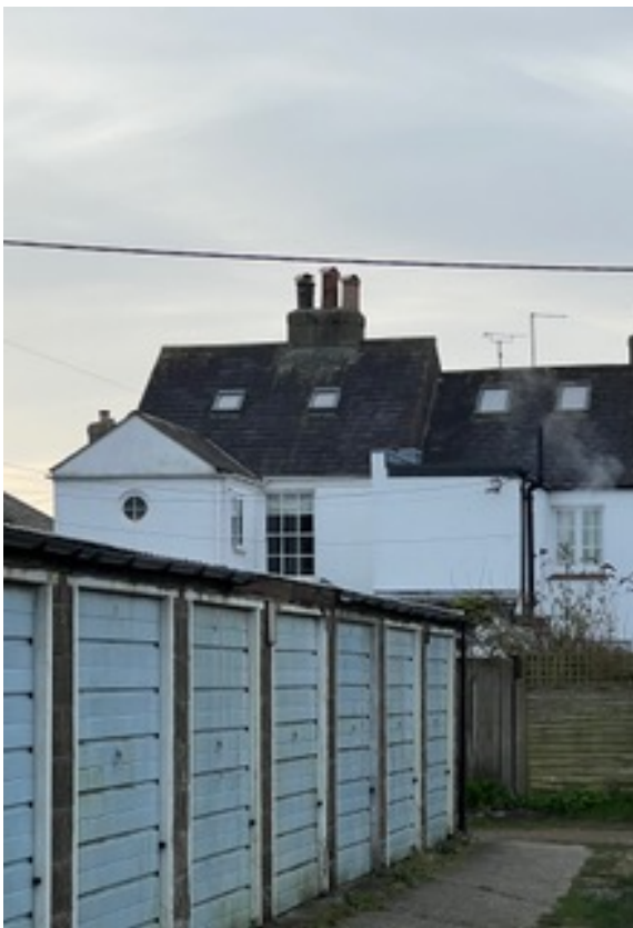
Fig. 9 – Round window on rear extension of property on North Road
