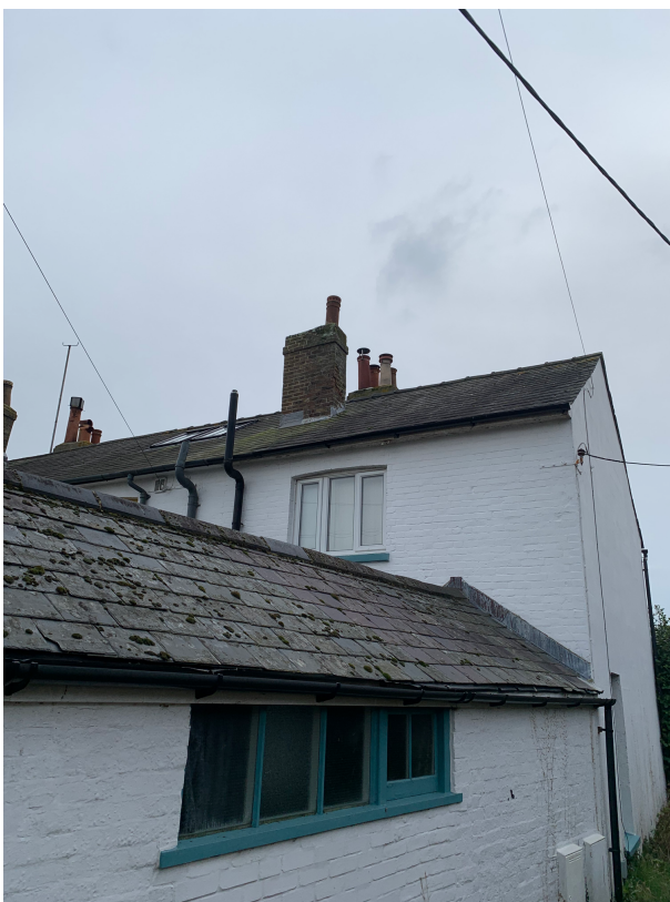
Fig. 6 - Rear view of house.
