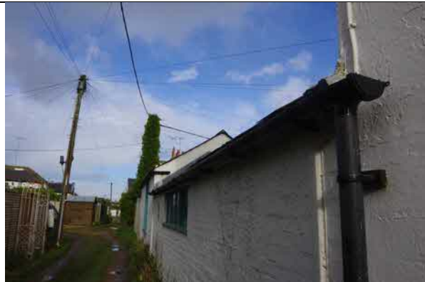
Rainwater runs at the left hand pitches of the extensions
