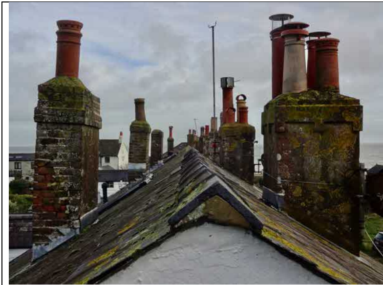
The chimney stacks
