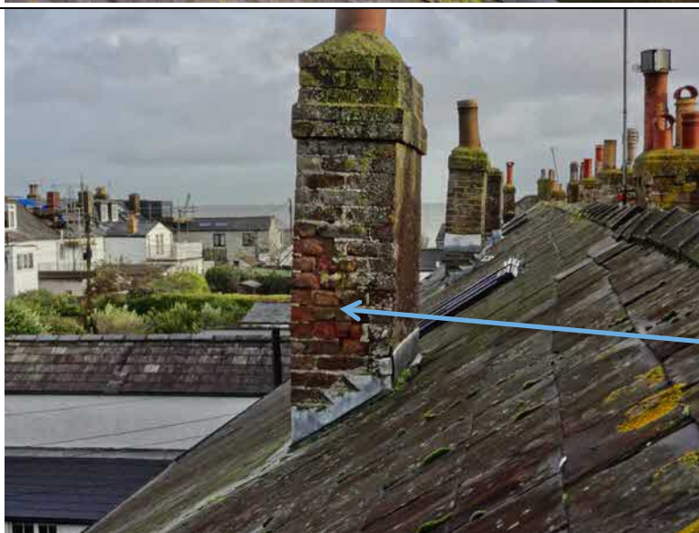
The rear stack
