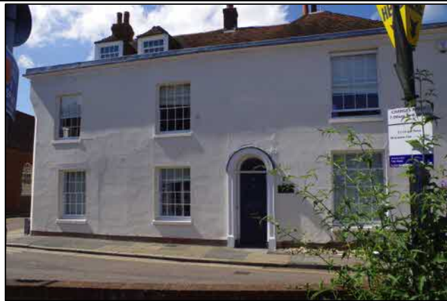
Example of localised repairs, including structural work; re-faced timber framed buildings
