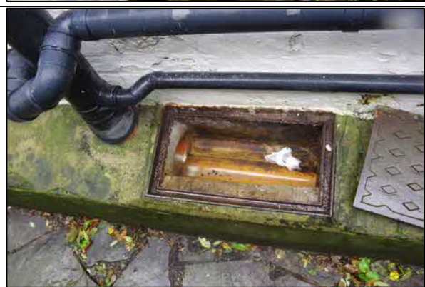
Inside the inspection chambers
