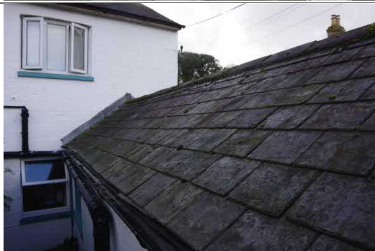
The right-hand pitch of the fi extension roof
