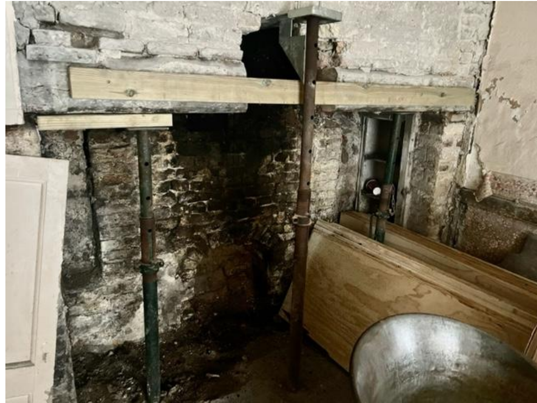
FIREPLACE (modern insert and brickwork removed exposing original)
