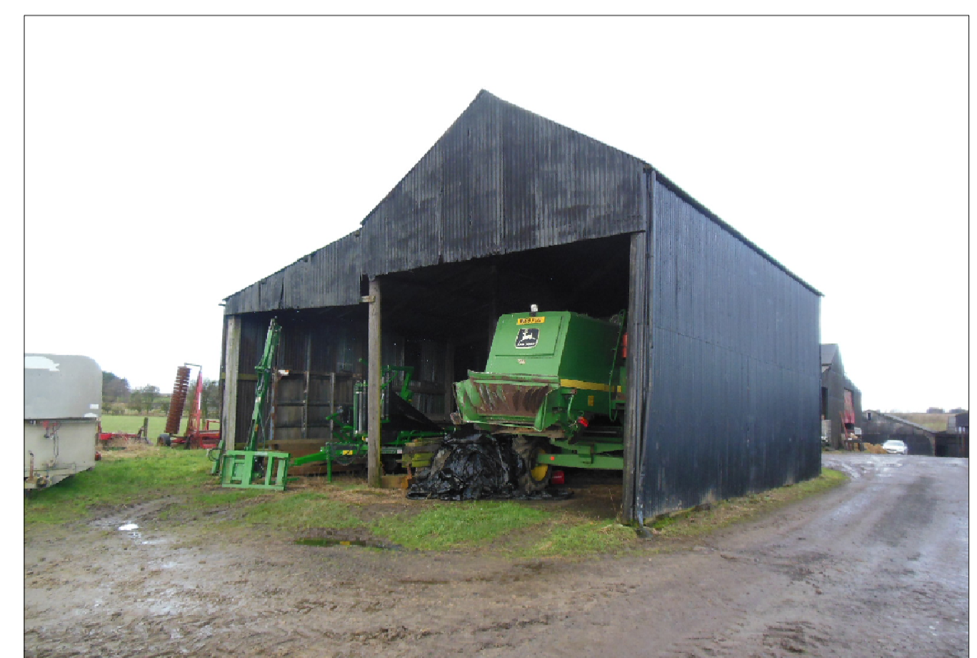
Existing shed to be removed
