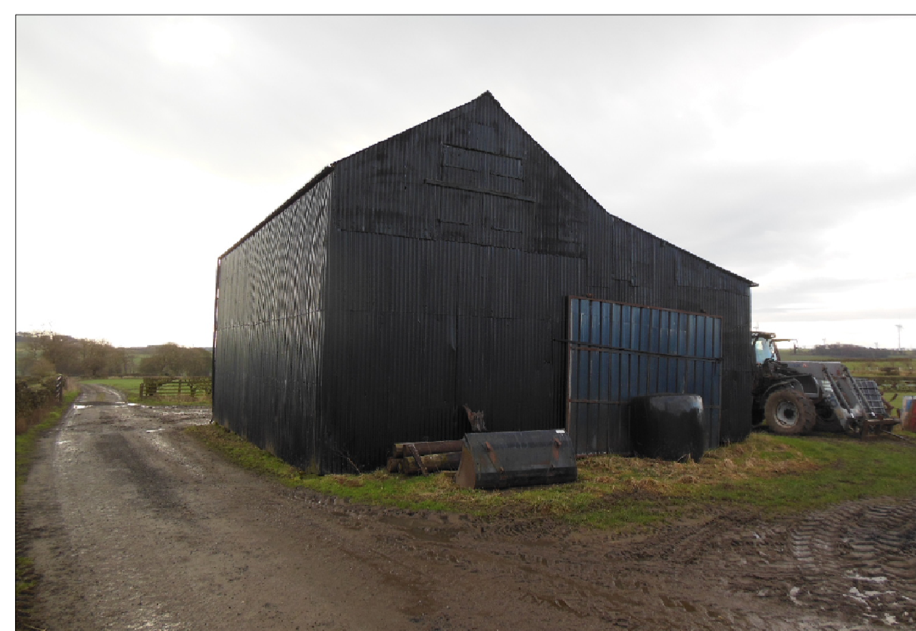
Existing shed to be removed
