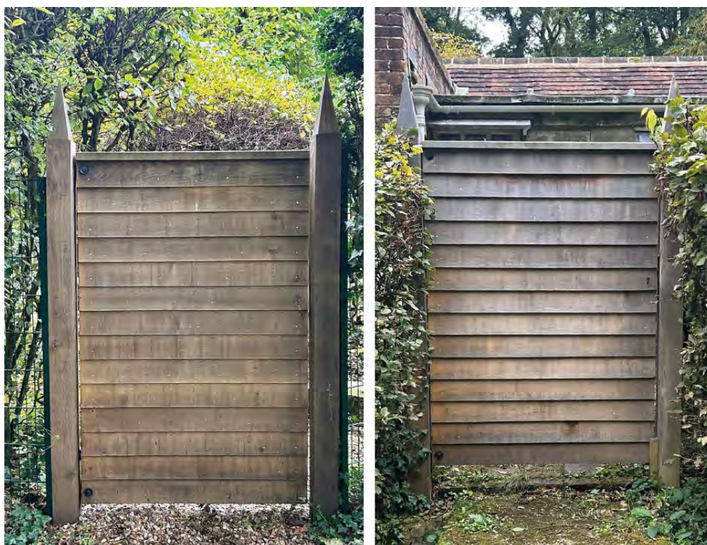
Figure 22. The gate to the kitchen (02) now offers privacy from passersby looking into the house and deer from jumping in.
