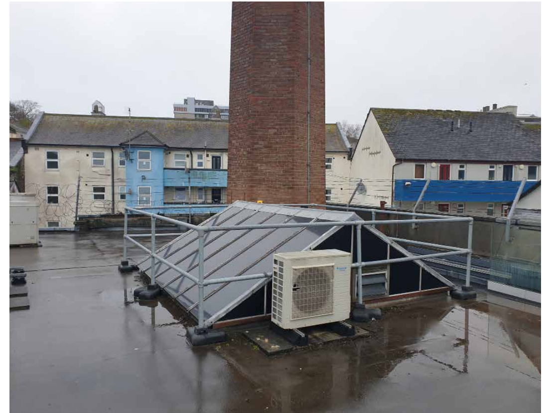
Fig 04 – Plymouth Gin Chimney and adjacent roof
