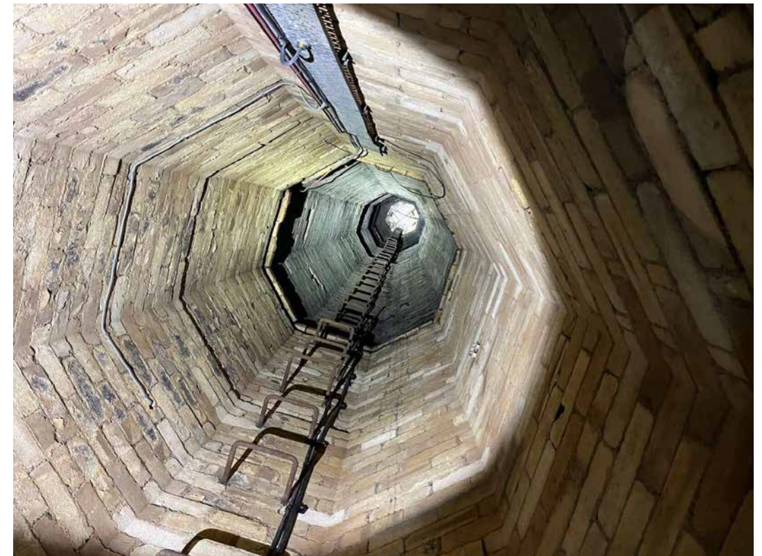
Fig 06 – Plymouth Gin Chimney internal view
